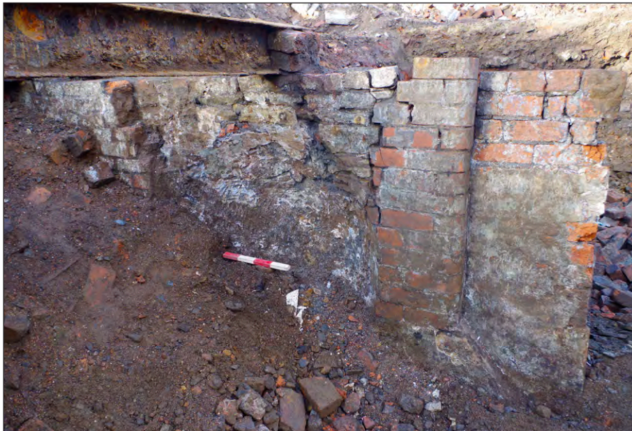
Plate 30: Wall 4019 with apsidal recess and environs from south-east
