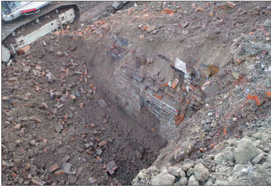
Plate 37: Structure 4354 seen under watching brief conditions from north-east
