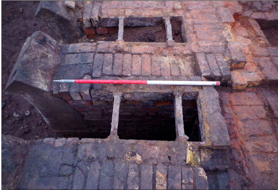
Plate 57: Example of melting hole bars in crucible furnace 4200 from east
