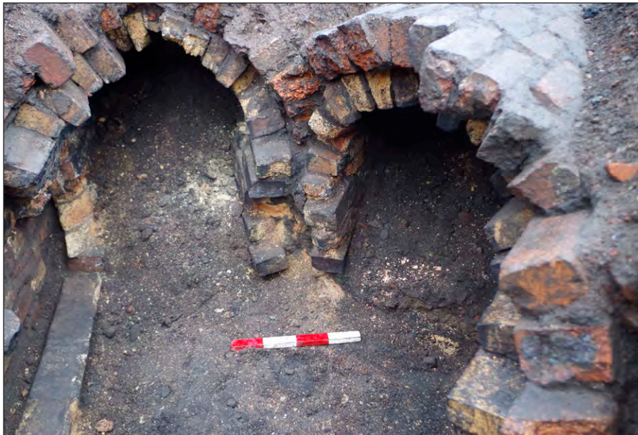
Plate 20: Flue 4104 splits. From east
