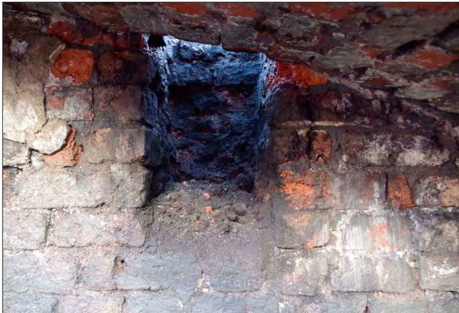
Plate 28: Small chimney 4070 under arch 1021 from west
