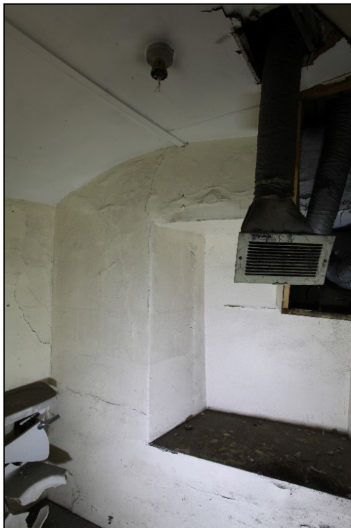
Plate 46. Overview of toilet cubicle with blocked window opening, facing south-east
