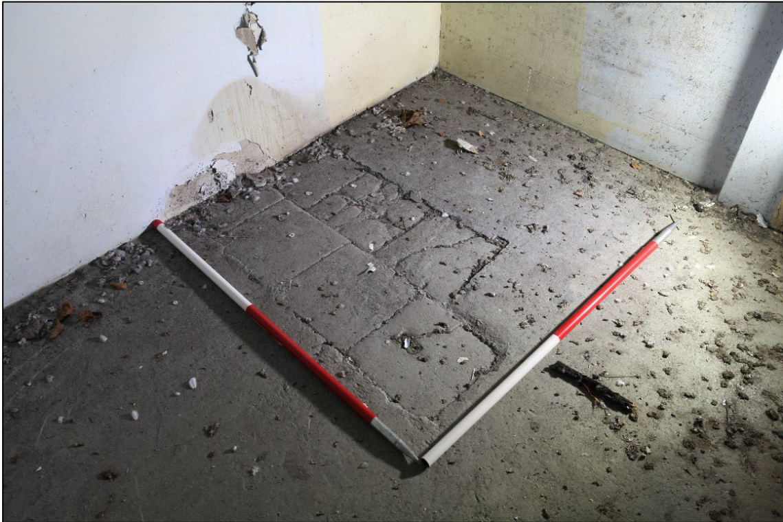
Plate 35. Detail of possible earlier stair support, facing south-east
