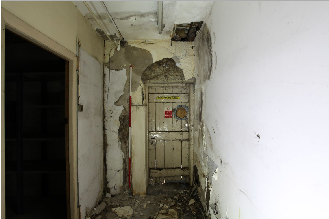
Plate 27. View along corridor, facing east
