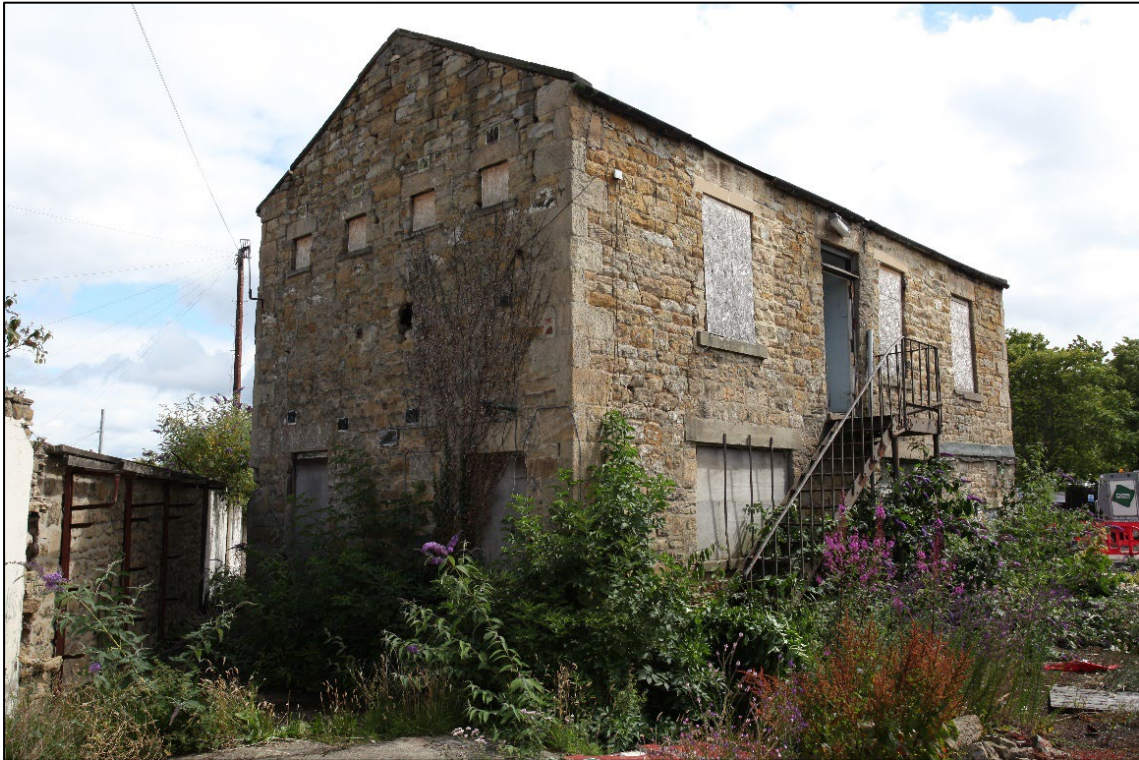
Plate 1. North and west elevations of the Fever Ward Building
