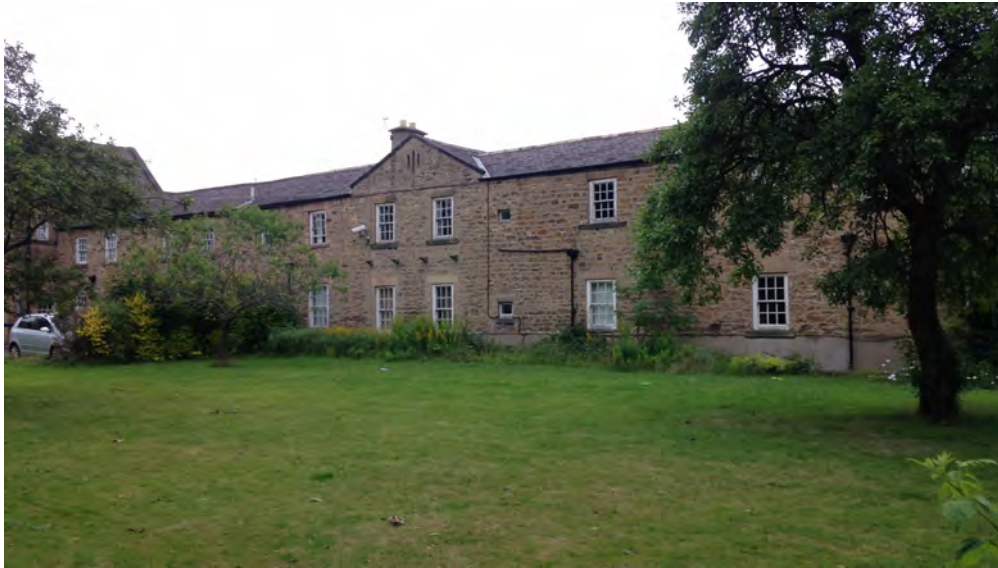
Plate 1: North-west facing view of the former Workhouse, now ancillary hospital buildings, to the west of the study site
