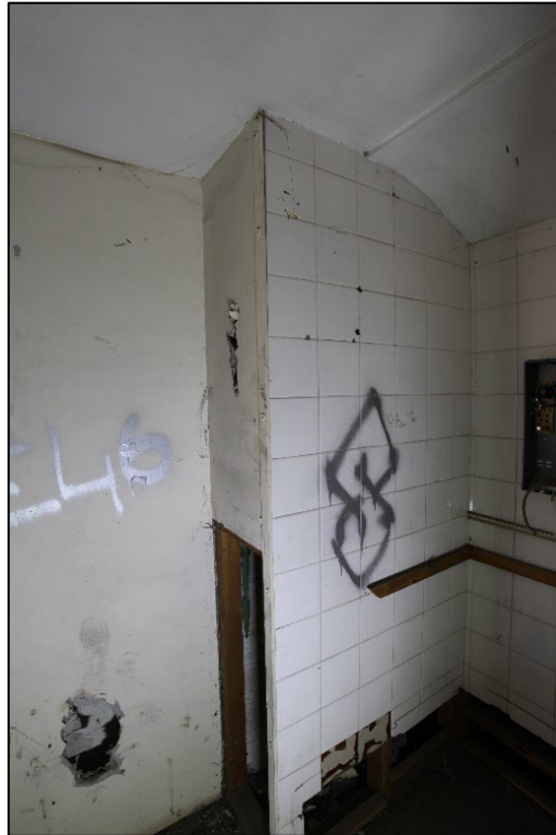
Plate 43. Overview of shower, facing north-east
