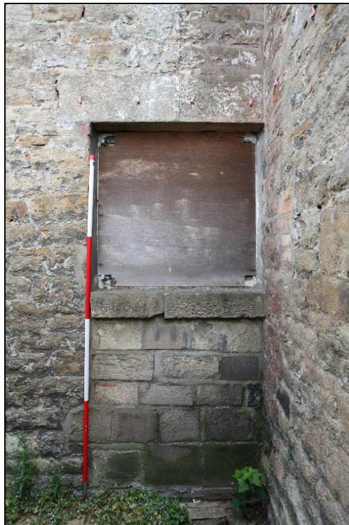
Plate 10. Window within blocked doorway to the north elevation of setback range
