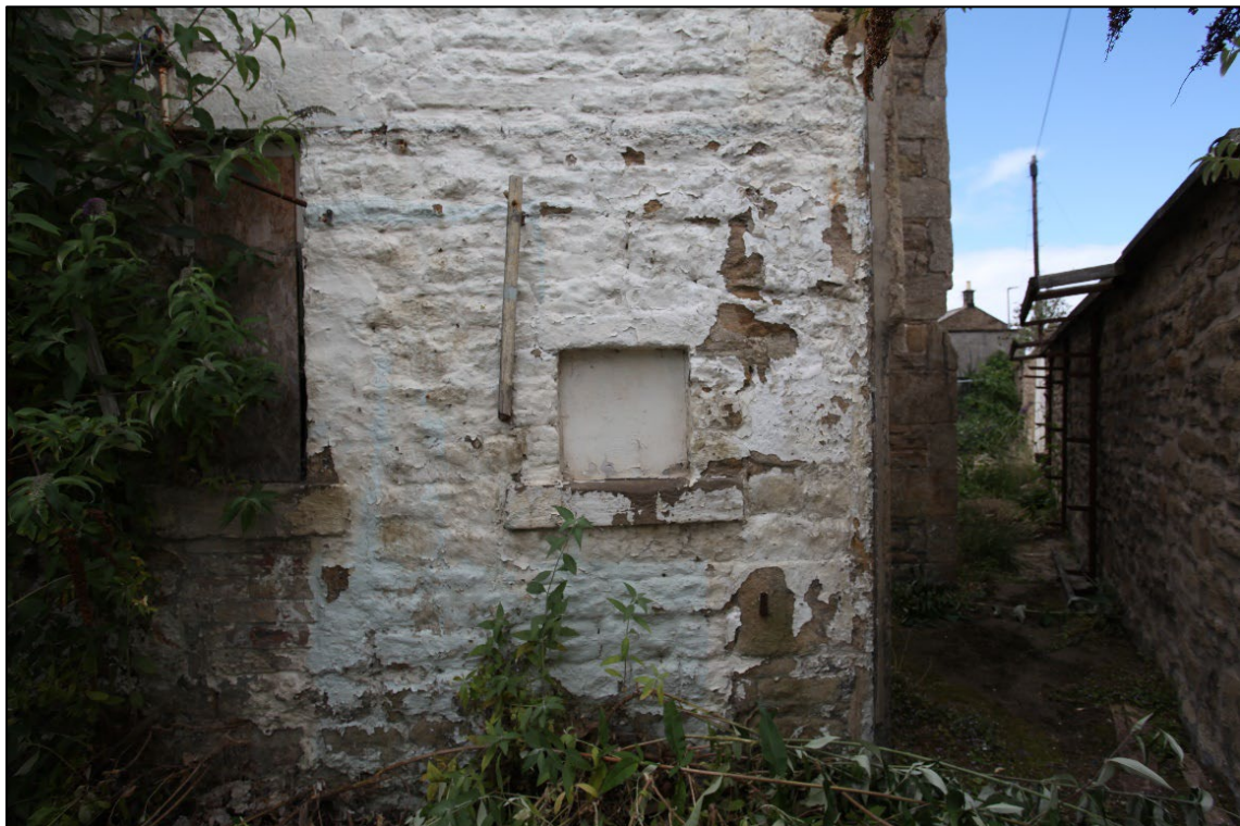
Plate 16. Original windows to the building's eastern elevation
