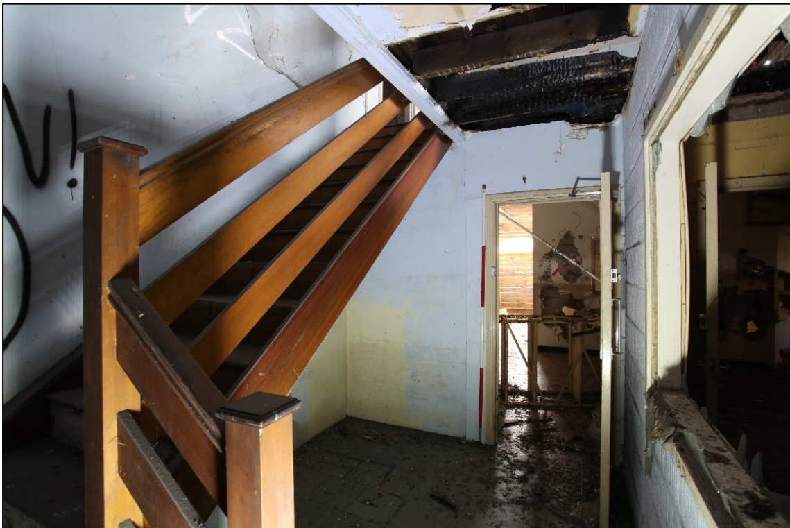
Plate 34. The staircase, facing south-east
