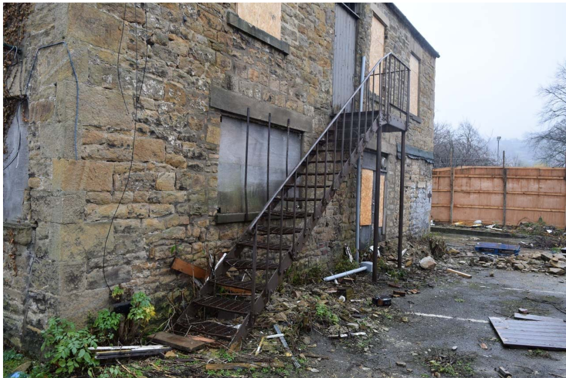
Appendix 3d: Detail of fire escape staircase on west elevation
