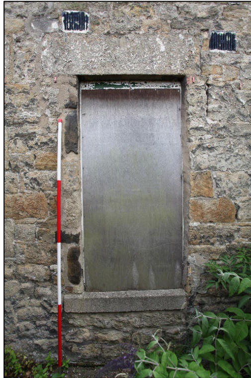
Plate 7. Eastern window within the northern elevation of the main block of the building – note the altered jamb and inserted sill.
