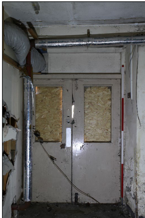
Plate 20. Double-width doorway to lobby, facing west
