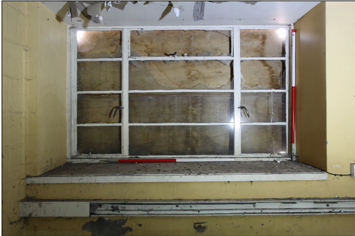
Plate 25. Detail of crittall window to room 3, facing west
