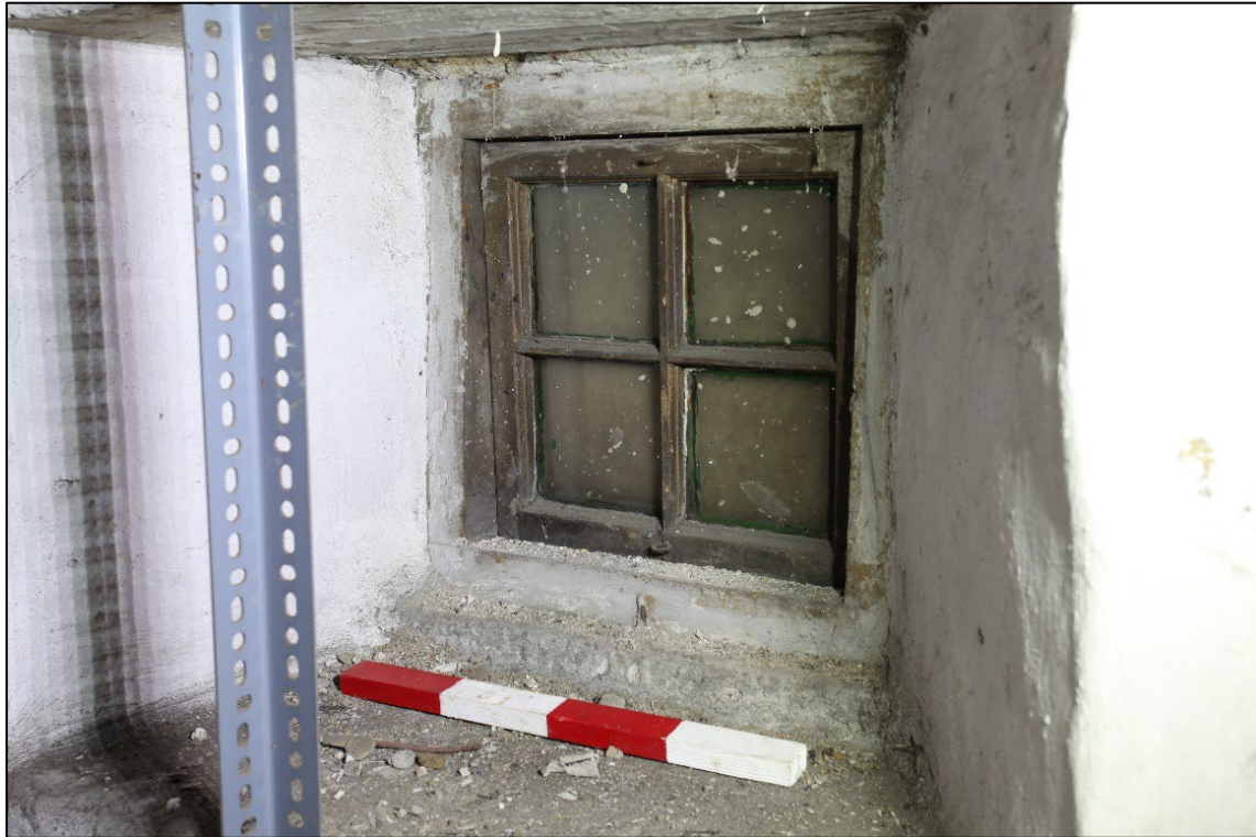
Plate 29. Detail of small four-pane timber casement in room 4, facing north-east
