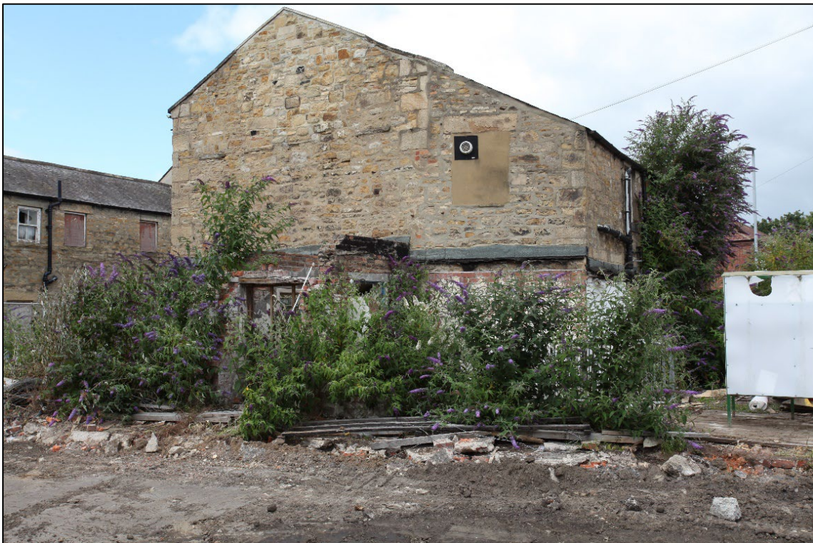
Plate 2. South and east elevations of the Fever Ward Building
