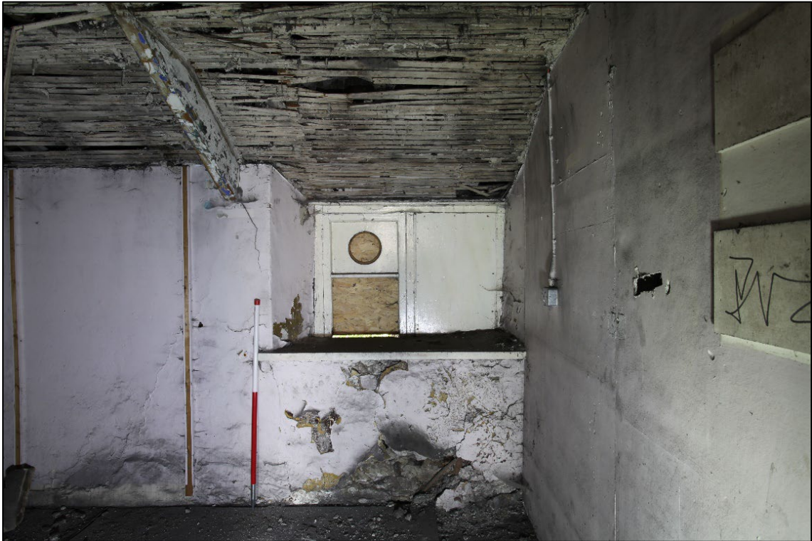
Plate 41. Detail of east window to room 7, facing east
