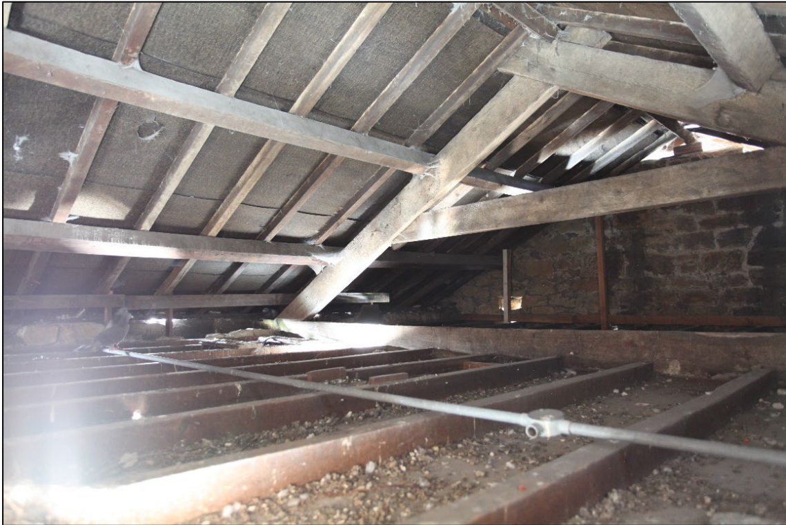
Plate 47. Overview of roof space, as seen through loft hatch, facing north-west
