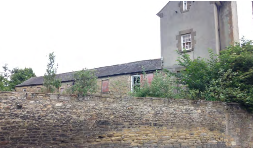
Plate 7: South-west facing view of the early 19th century Workhouse buildings
