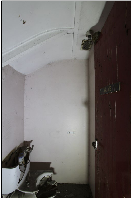
Plate 45. Overview of toilet cubicle, facing south
