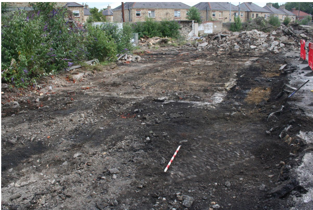
Plate 52: Trench 1 from the south-west showing structures 103 and 104
