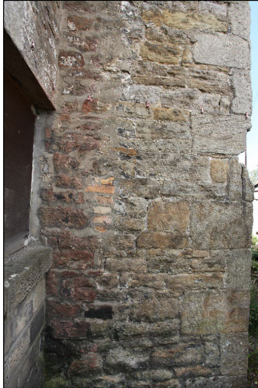
Plate 13. Variation to blockwork at the intersection of the main block and set-back range – possibly related to a removed chimney stack
