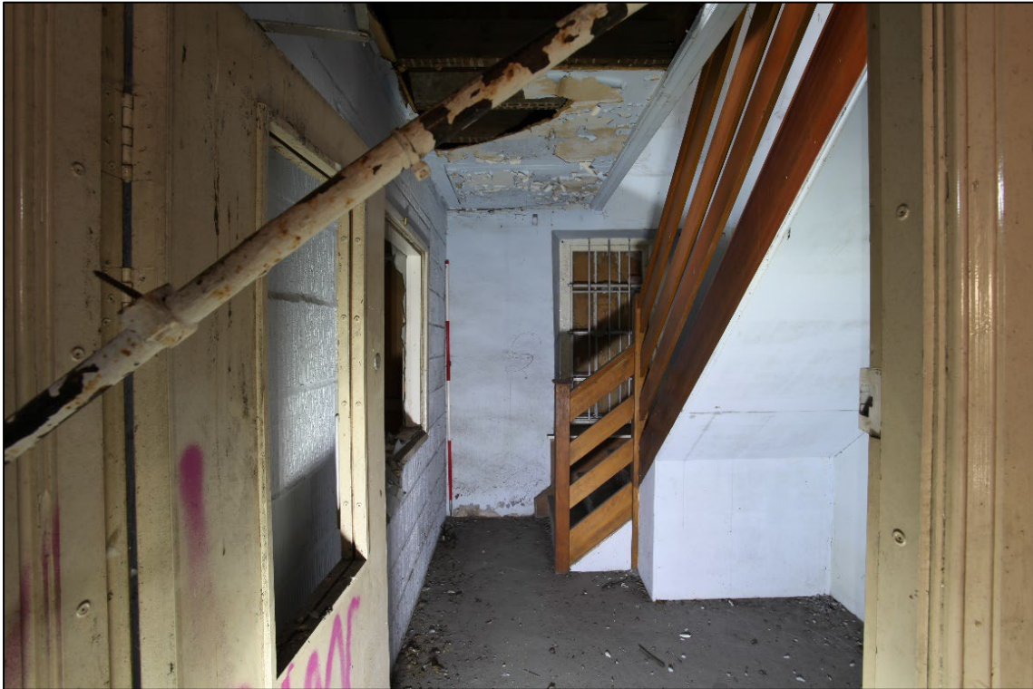
Plate 33. Overview of staircase room, facing north
