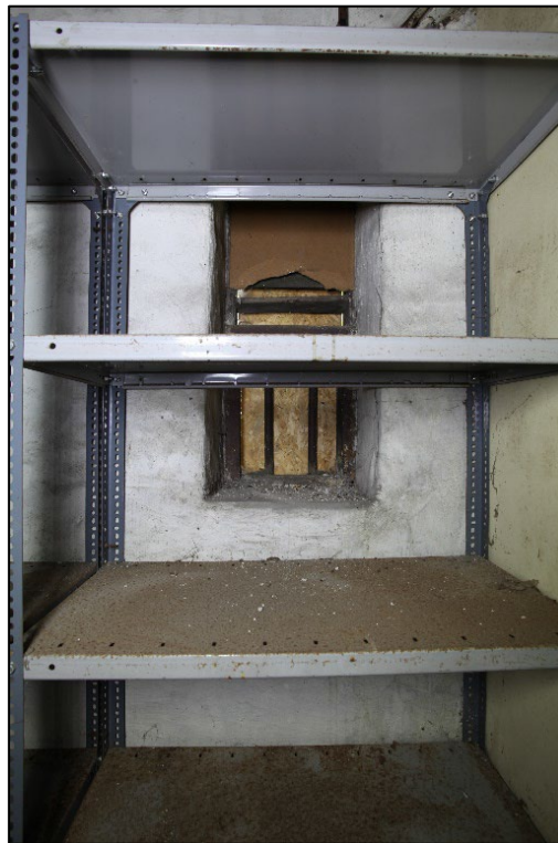
Plate 30. Detail of louvred and barred window opening in room 4, facing east
