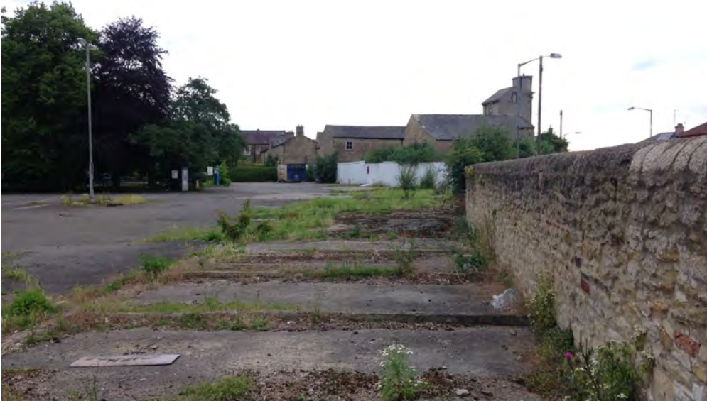
Plate 5: Footings and hardstanding remains of buildings evident within the north-east corner of the study site
