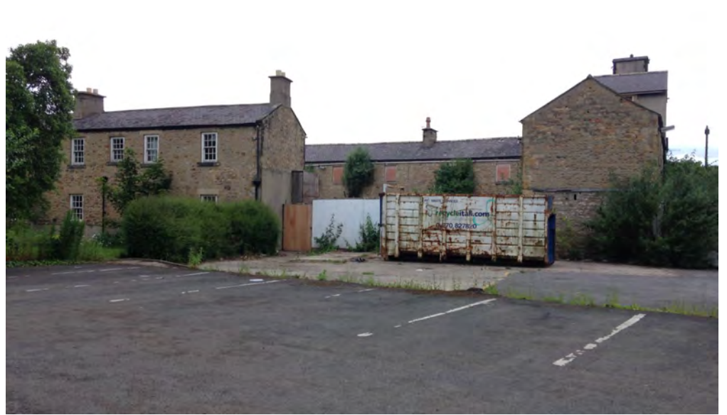
Plate 8: North-west-facing view of the former Workhouse buildings in the north-west corner
