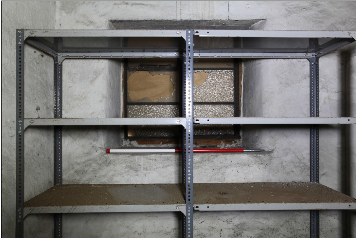
Plate 31. Detail of inserted crittall window in room 4, facing north
