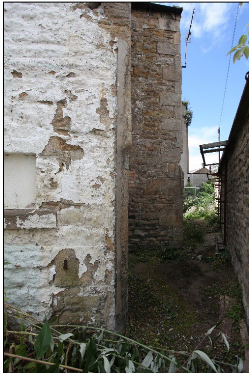
Plate 12. Bullnosed blockwork to the eastern corner of the northern elevation, facing west
