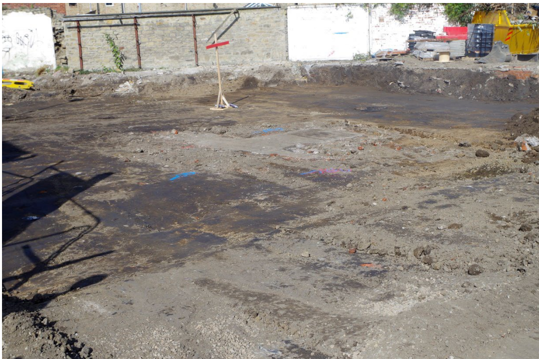
Plate 62: Trench 2 upon completion of excavation, taken from the south-south-west
