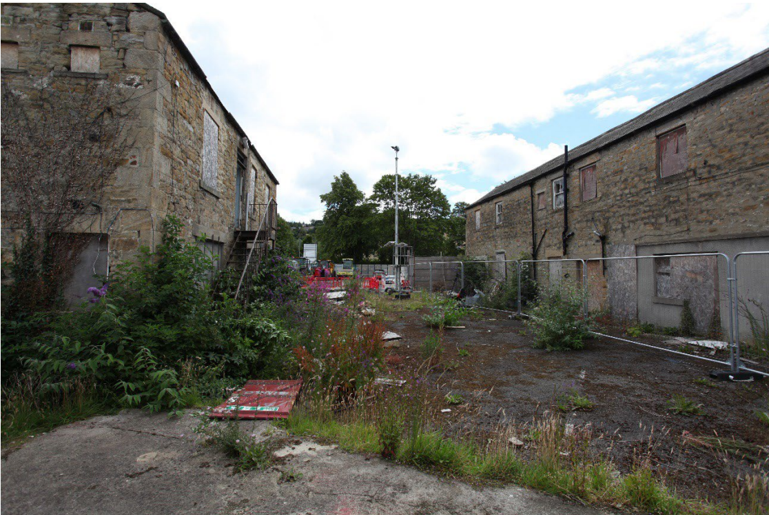
Plate 48. View south across the west of the Site, seeing the Fever Ward building (left) as it relates to the former Hexham Workhouse
