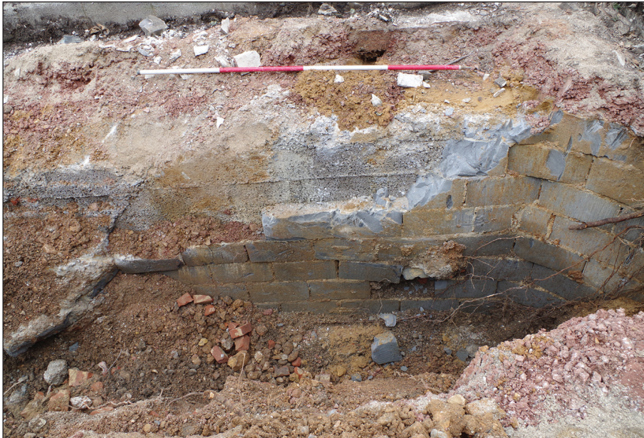
Plate 2: South facing section of retaining wall
