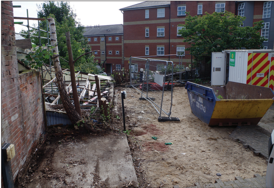
Plate 1: Pre-works site conditions, view from the west
