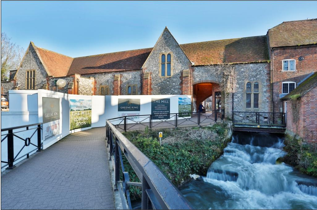
Plate 7: East end of south elevation showing new walkway arch, originally a double lancet window
