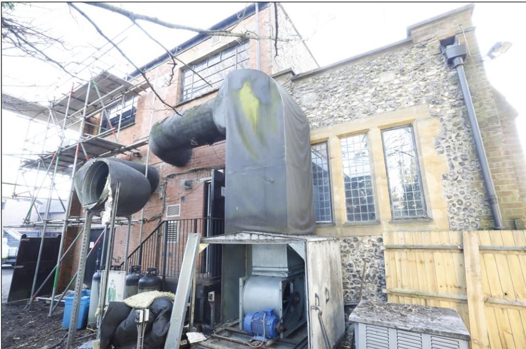
Plate 2: West end of building showing flint and stone façade construction against brick
