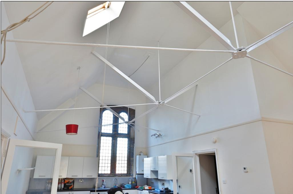
Plate 12: Iron roof trusses and tie rods above north buildings
