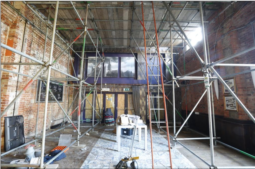
Plate 8: Interior of original Generator Hall viewed from west showing inserted glazed entrance wall
