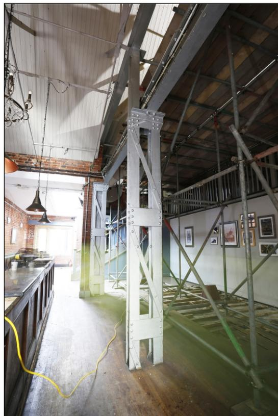
Plate 10: West end of Generating Hall showing riveted stanchions and upper rail of travelling crane
