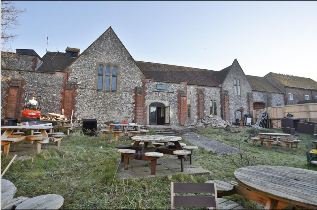
Plate 1: South facing elevation showing flint and stone walls and lancet windows
