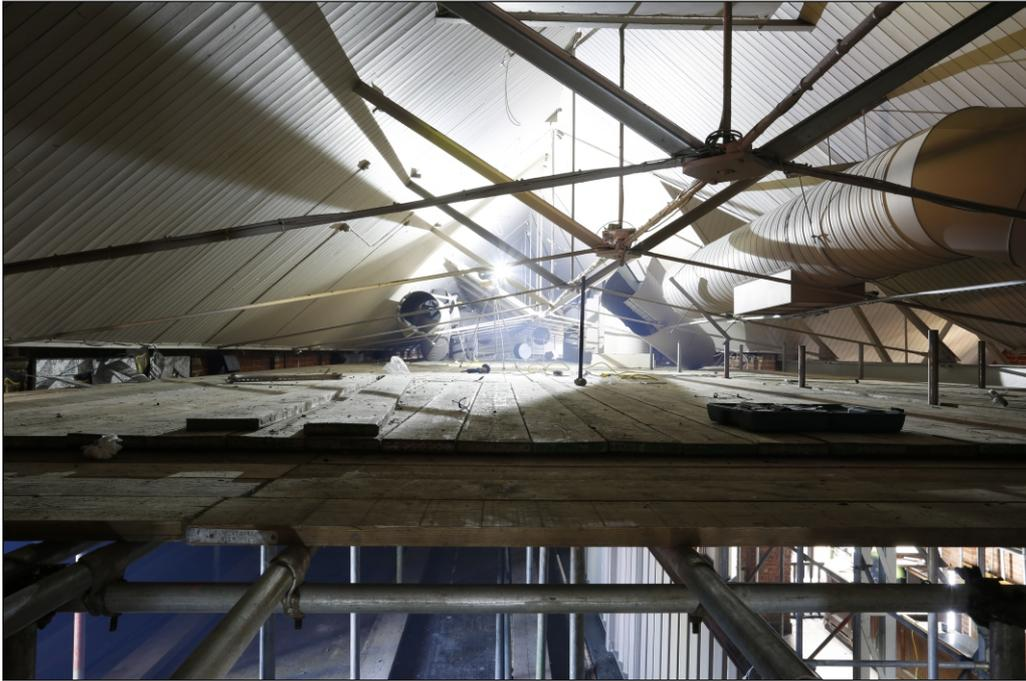
Plate 11: Iron roof trusses above working platform in Generating Hall
