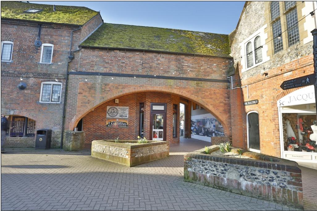
Plate 5: North side of east end showing original wide brick arch (once internal)
