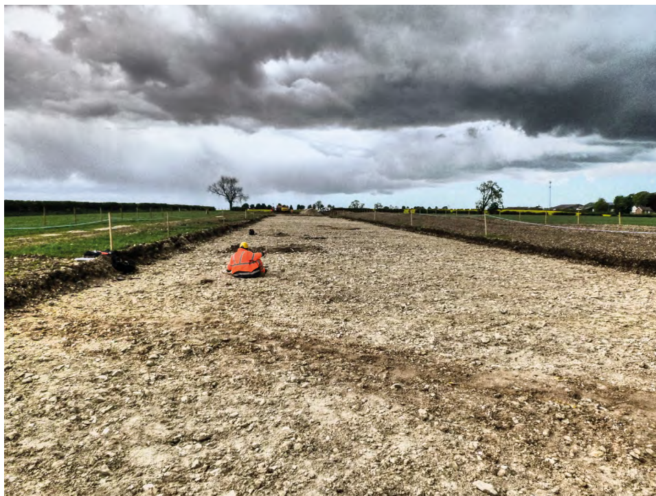
Figure 4.14 The view northwards along the Pitchmoor site
