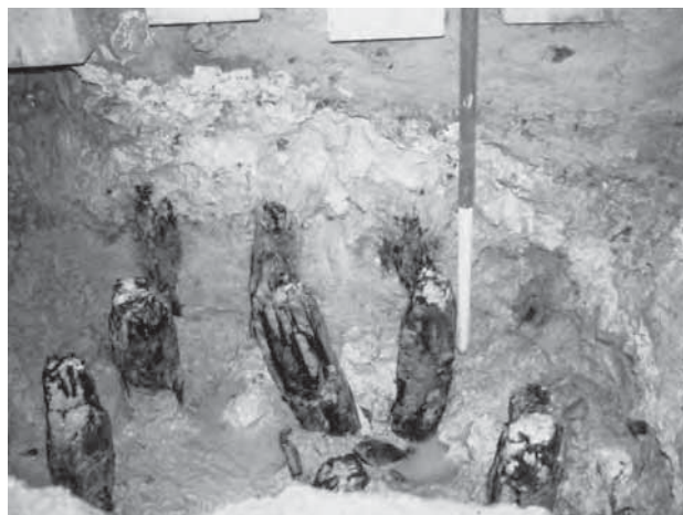
Plate 2.1 Wooden piles driven into the natural that formed part of the foundations of the Roman fort wall, revealed at the bottom of Trench 2. See Figure 2.1 for section drawing
