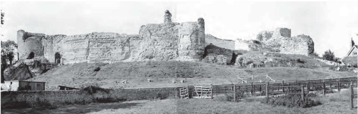
Plate 1.5 Photograph of Pevensey Castle from the south east, taken c. 1930, following the removal of the mound that covered the Keep by the Ministry of Works, revealing the interior of the Keep. The South Tower and postern gate of the Inner Bailey lies on the far left, and the East Tower on the far right. The Roman bastion at the centre of the photograph was used as the Keep's South East Tower, to the north (right) of which the Roman fortress/medieval keep wall has collapsed (© Crown Copyright, NMR)
