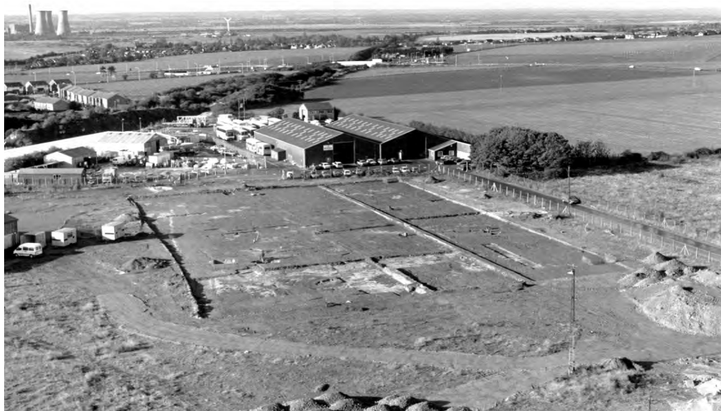
Plate 4.1 Manston Road, Ramsgate: General view of excavation looking south
