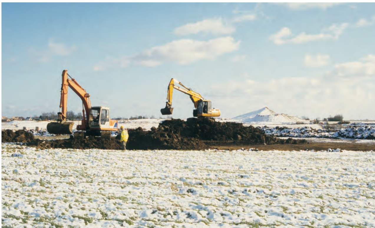
Plate 3 Topsoil stripping at Lower Cambourne in winter
