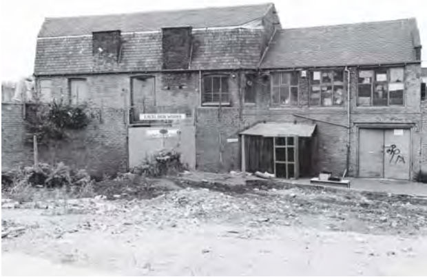
Figure 32 Hoyle Street Works, south-west elevation of buildings B1 and B2
