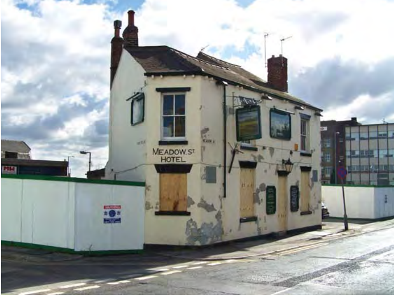
Figure 58 The Meadow Street Hotel, viewed from the west
