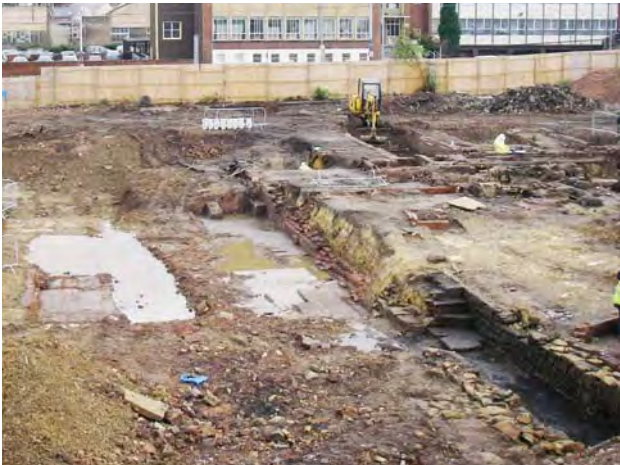
Figure 23 Hoyle Street Works north-east range, viewed from the north-west
