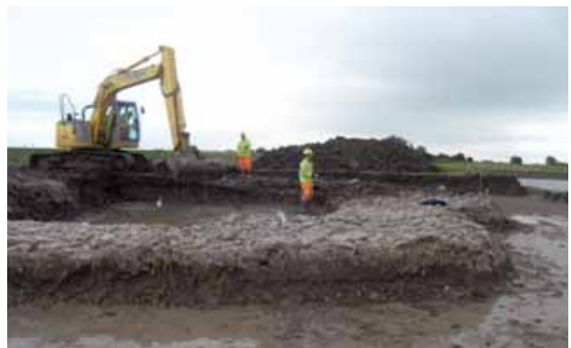
Plate 2.14 Pond 21437 and cobbled surface 21422 under excavation
