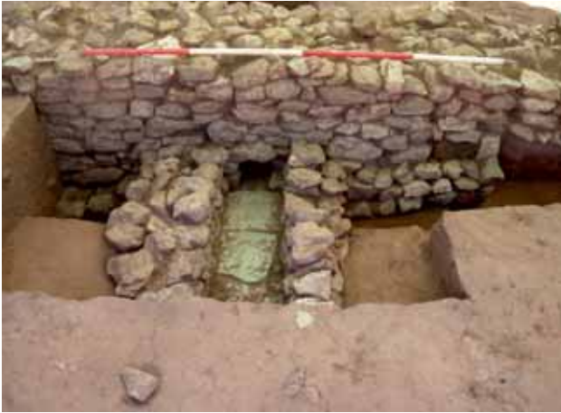
Plate 3.11 Drain 10071 within ancillary building/Room 10; south wall 10040 (note shallower wall foundations to right), from north
