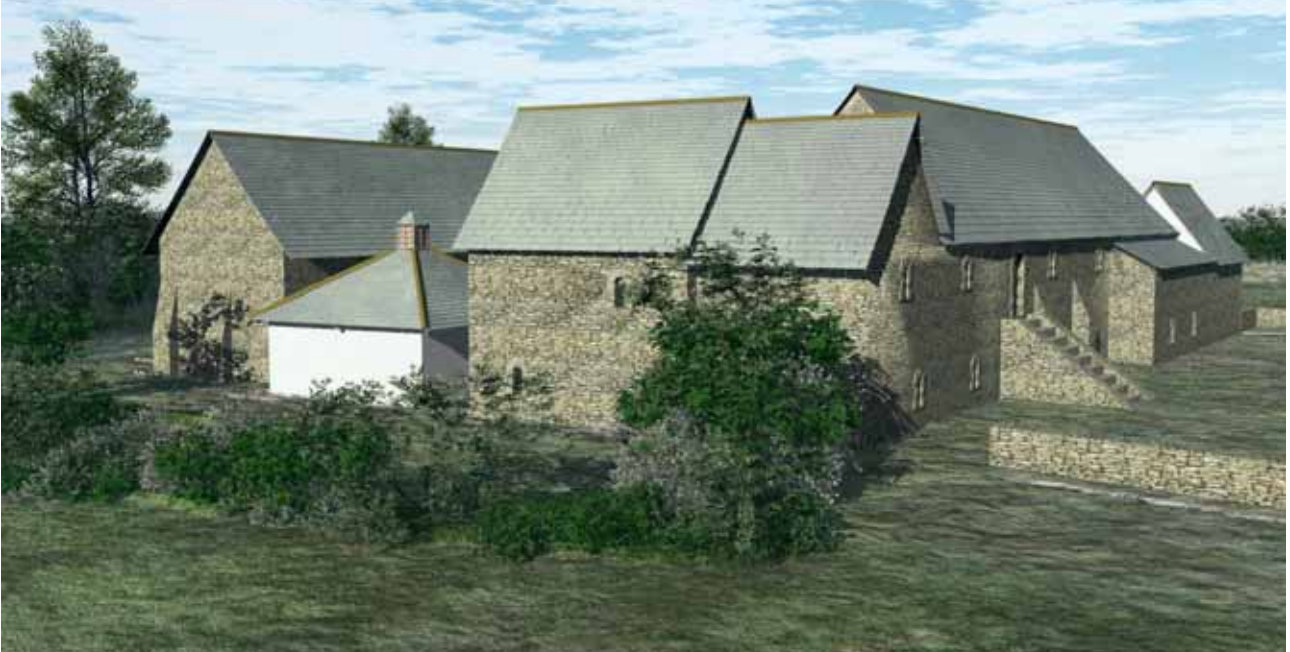
Figure 7.1 Visualisation of north elevation of manor house, service range, detached kitchen and east end of ancillary building, from north-east
