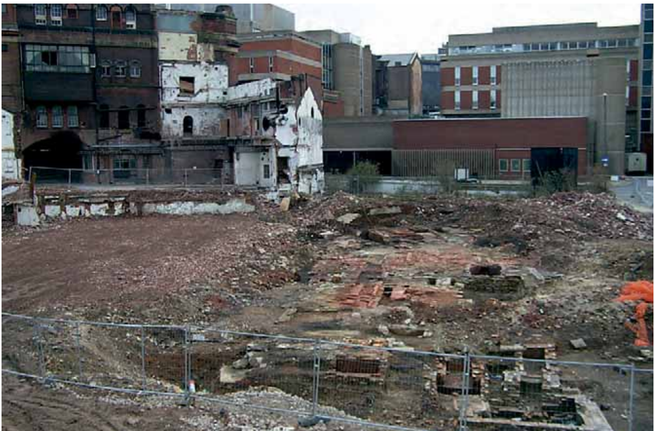
Plate 1 Remains of Marshall's cementation furnaces (prior to preservation in situ), with retained brewery buildings top left (view from north) (© University of Sheffield. Reproduced by permission)
