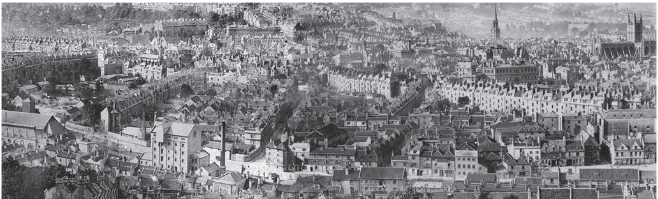
Plate 5.1 Panorama of the Avon Street district, from the south, taken between 1880 and 1885 © B&NES Council
