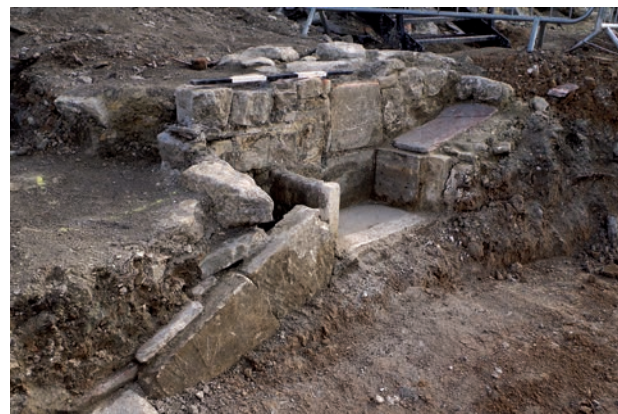
Plate 4.11 Late 18th-early 19th-century drain to the rear of 13 New Quay (B11), incorporating a sewer gas trap, view from the west
