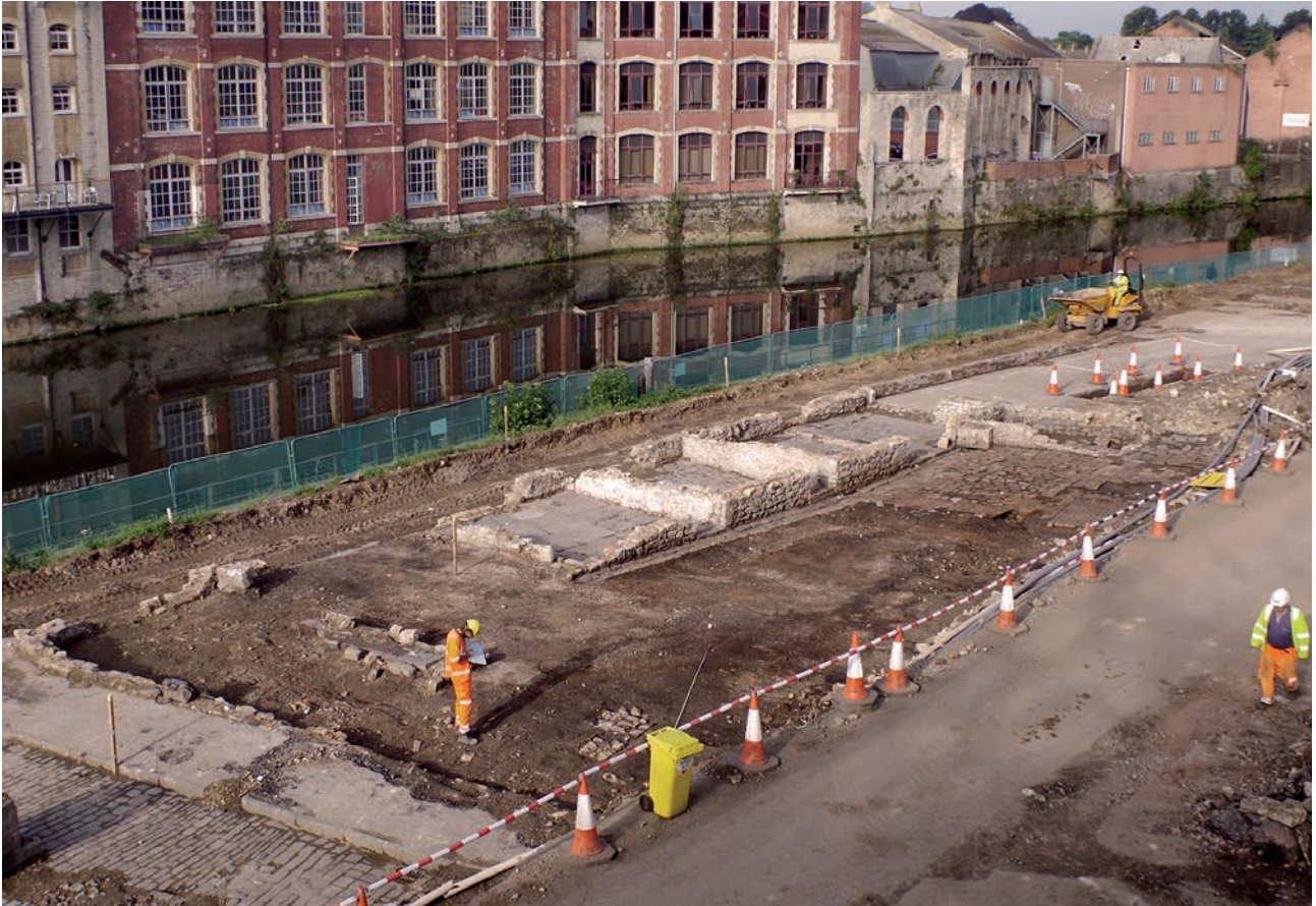
Plate 5.4 Commercial stables (B33, B34 and OA28) at the southern end of Avon Street, view from the north-east, with the Albion Stay Factory and the Newark Works in the background
