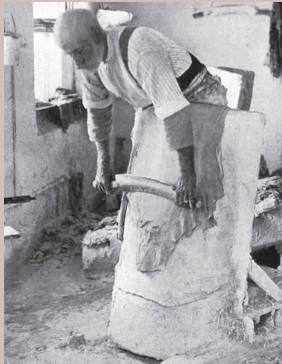
Plate 4.25 Working sheepskins on a 'beam' to remove fat and lime. Image of the Homewell Parchment Works, Havant, published in The Sphere, 28 September 1928, 208 © Mary Evans Picture Library
