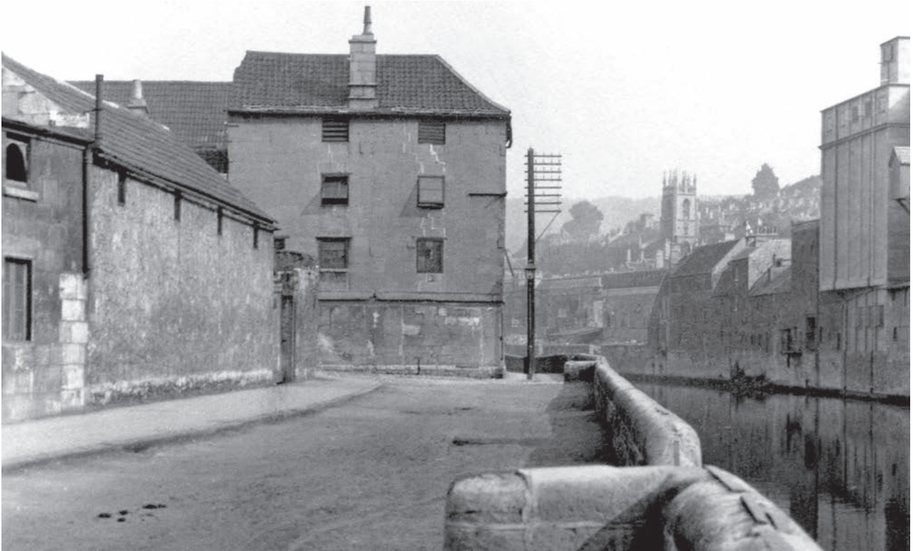
Plate 4.37 c. 1930 view of New Quay, from the north-west, showing late 18th-century warehouse B7 (centre) and c. 1874 stable B33 (left) © B&NES Council
