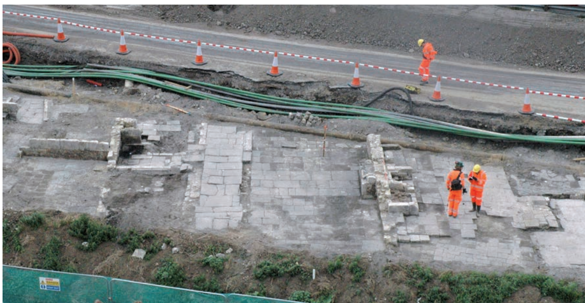
The Duke of York public house, 4 New Quay (B16), from the south (see Chapter 4, B16–B17: Ward's Warehouse and the Duke of York public house and brewery, 4 New Quay)
