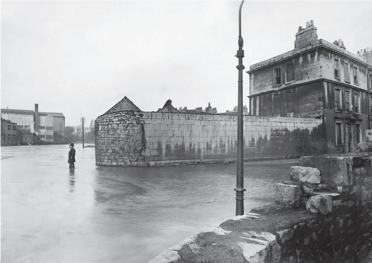
Plate 7.1 Flooding at the southern end of Avon Street on 27 February 1937, from the east, showing 49 Avon Street (constructed in the 1730s) and adjacent stables (B34), which were constructed c. 1874 © B&NES Council
