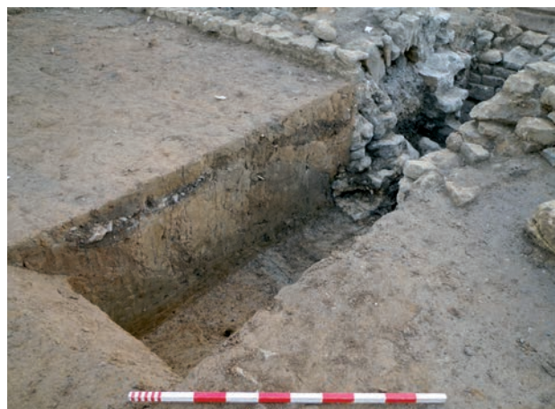
Plate 2.1 Section across the medieval ‘Fosse Dyke’ (S1), culvert S19 and wall S2, from the west
