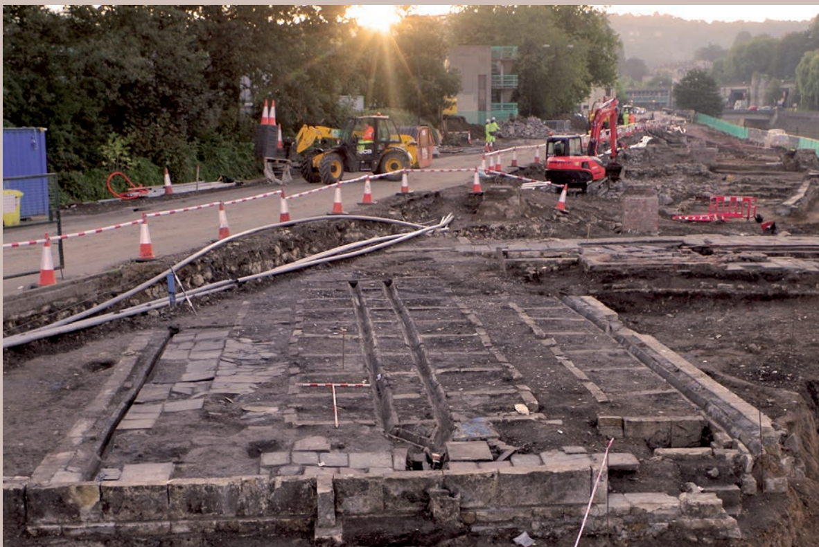
Plate 5.14 1853 laundry block, from the west
