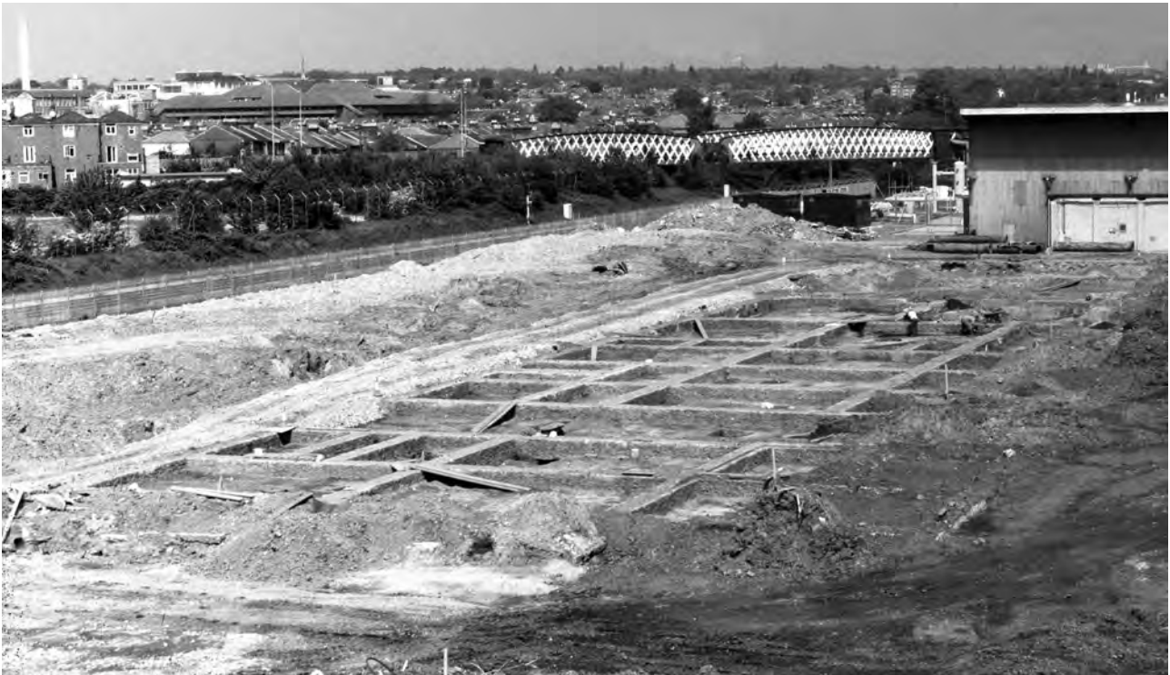
Figure 38 View of the West Stand excavation area, looking north-west, showing modern footings
