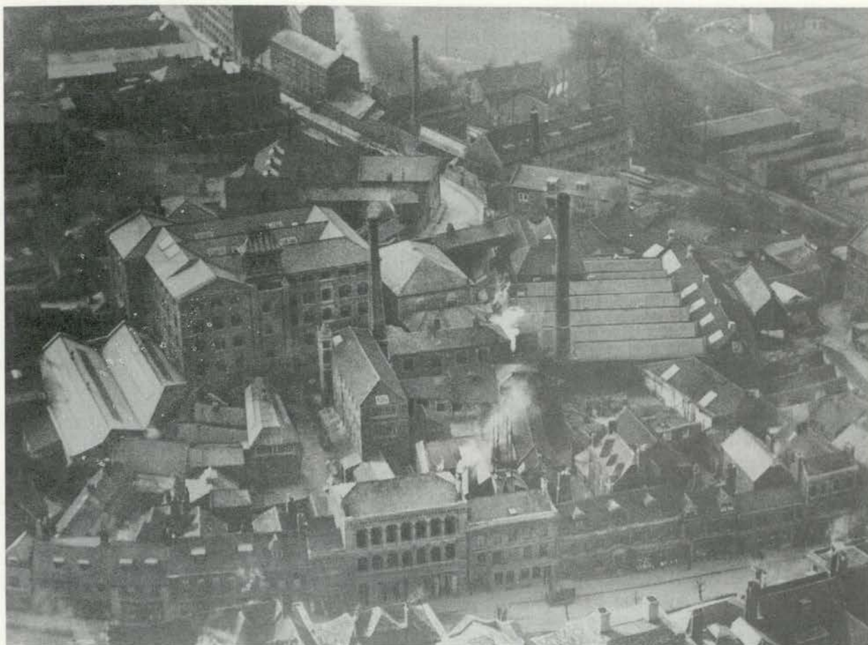
Plate 2 The Trowbridge woollen mills: aerial view from the north, c. 1928. This industrial landscape is dominated by Home Mills; the frontages of the buildings along the south side of Fore Street are at the bottom of the photograph
