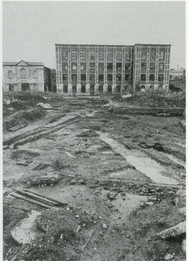
Plate 3 Home Mills and the Bethesda Chapel in 1988; viewed from the south with the area of the 1988 excavations in the foreground. Both buildings have been preserved within the modern redevelopment
