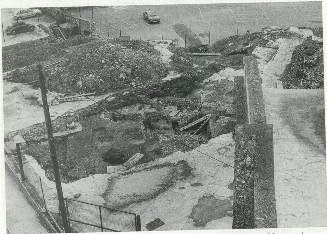
Plate 5 Excavation 1987: Trench C viewed from the east. The patch in the tarmac of the carpark immediately beyond the trench marks the position of W132
