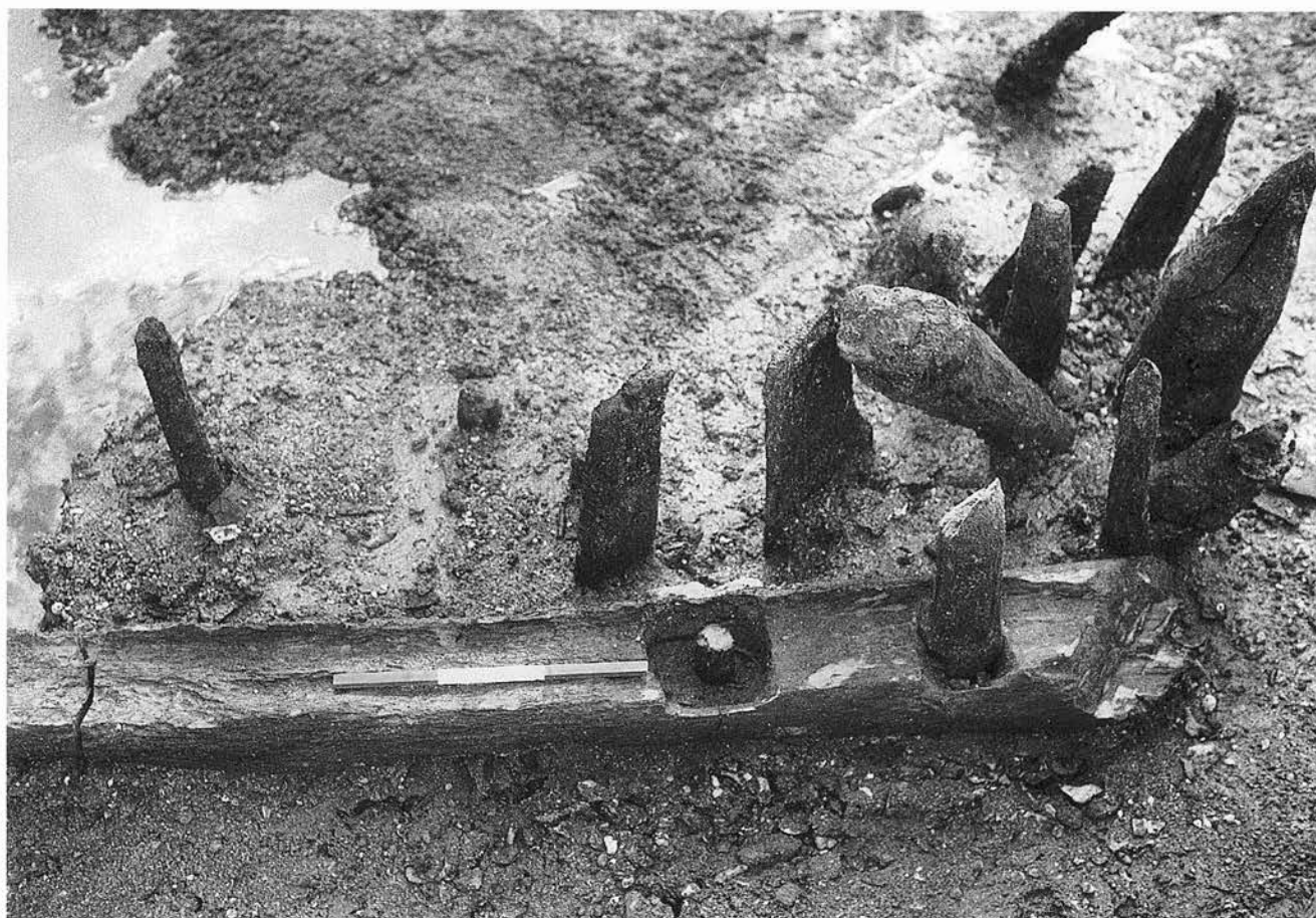
Plate 13 Anslow's Cottages: Timber structure 1594 (Phase 4b)
