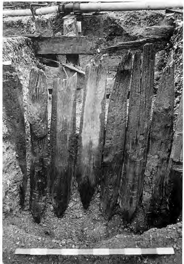
Plate 11 Abbey Wharf W61A: Phase 8 revetment
