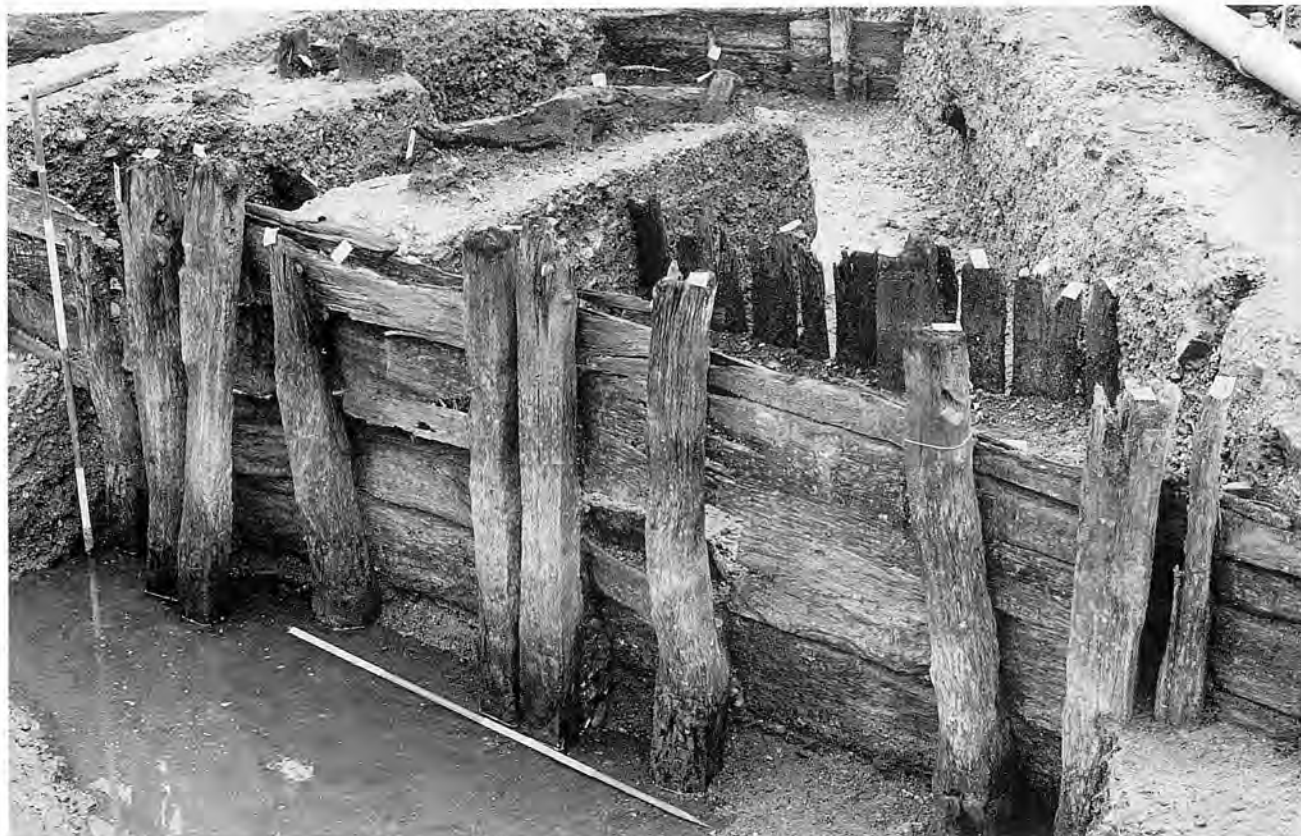
Plate 12 Abbey Wharf W61A: Phase 9 revetment
