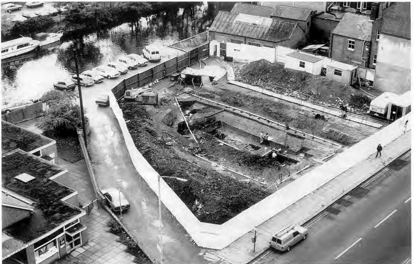
Plate 14 Crane Wharf: general view of excavations
