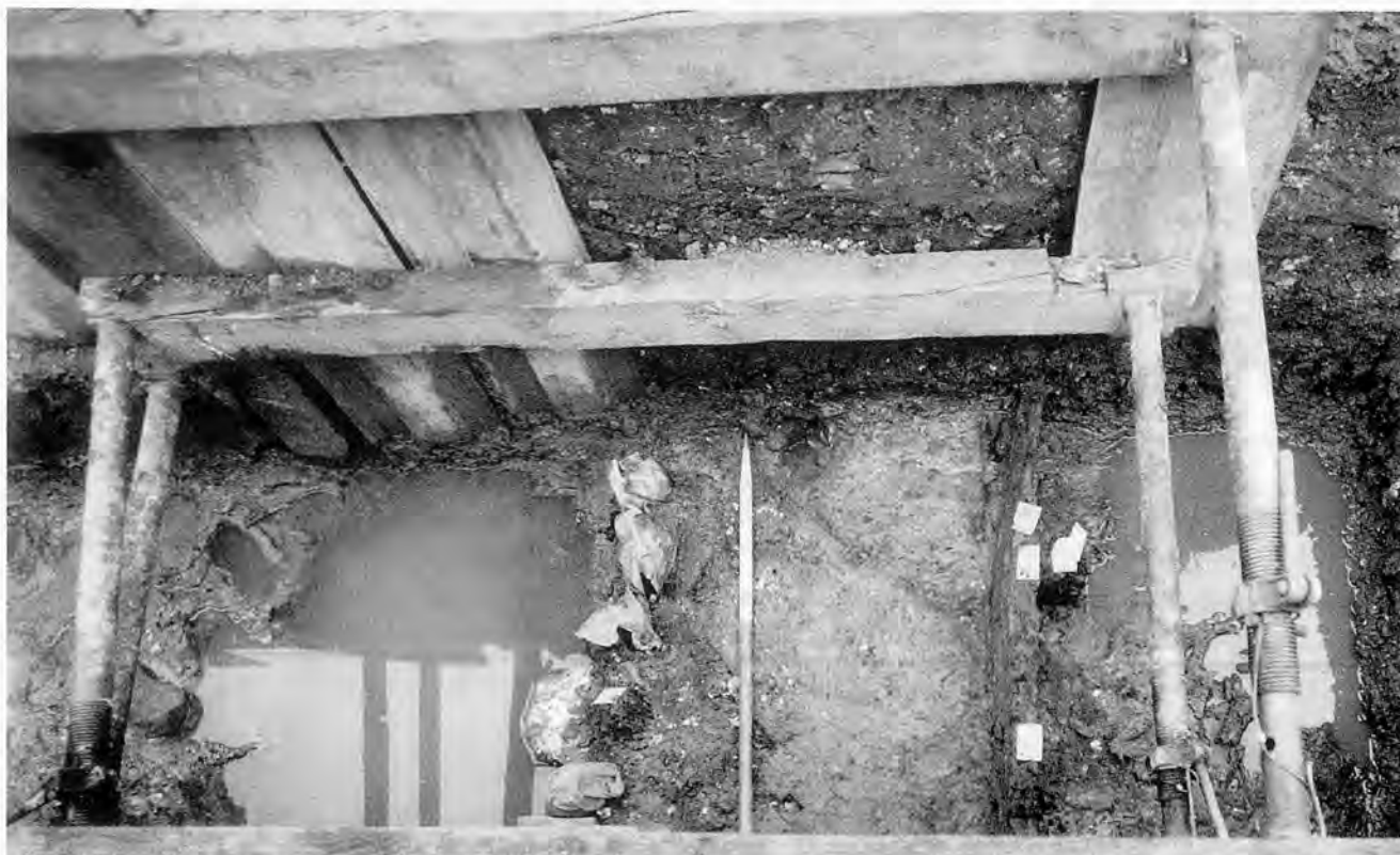
Plate 17 Fobney Street: excavation area
