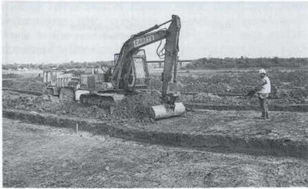
Plate 16 Colluvium excavation area during stripping, looking north-east towards the M4
