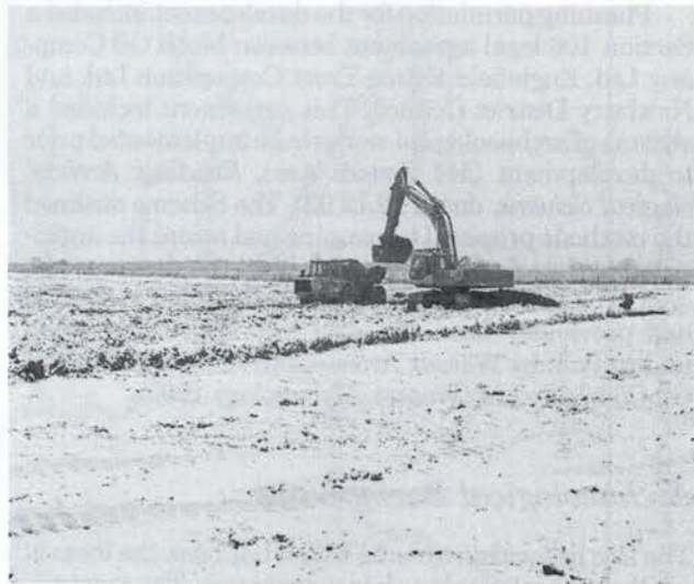
Plate 15 Foul weather conditions during topsoil stripping, looking south-west to Deans Copse
