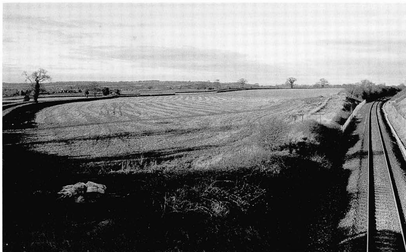
Plate 7 Castle Hill: view of the site from the north, from the old railway bridge, prior to excavation
