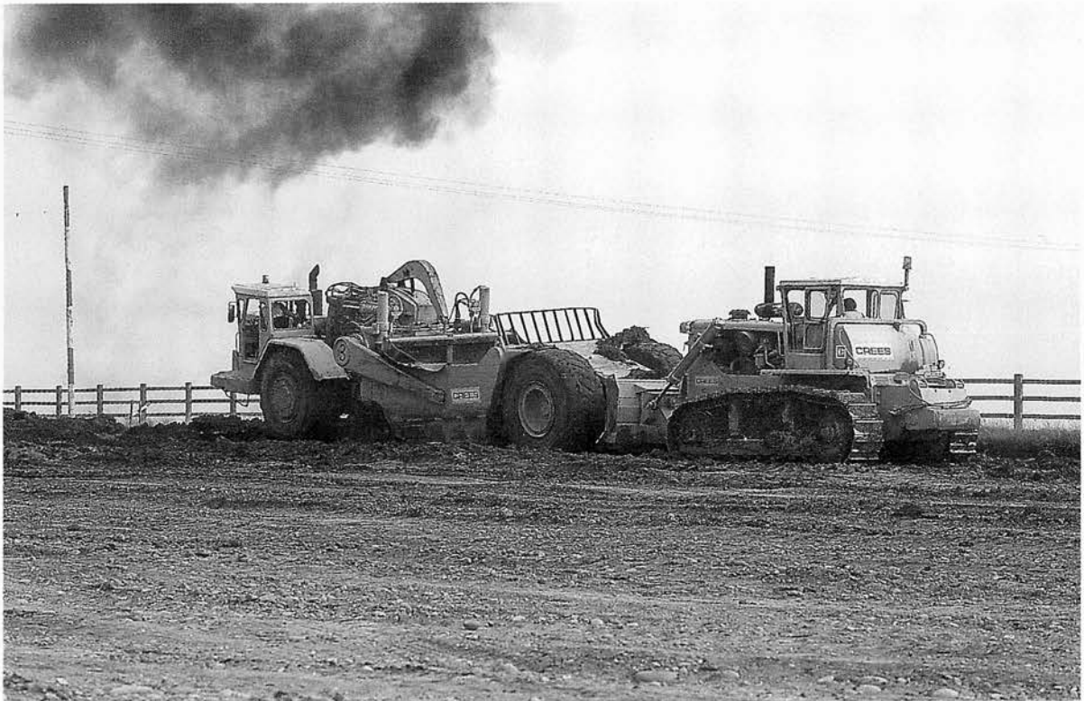
Plate 1 Topsoil stripping at Long Range
