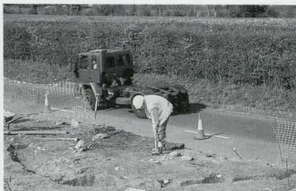
Plate 33 Pomeroy Wood: building 4103 viewed from the south-east illustrating the extent of truncation by the existing A30
