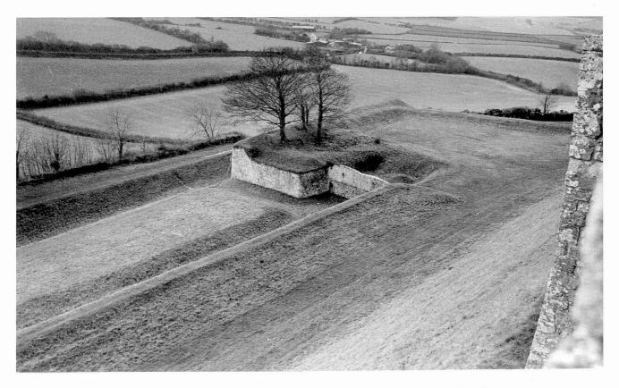
Plate 46 South bastion of the artillery fortress from the north-east showing east flanker and orillon
