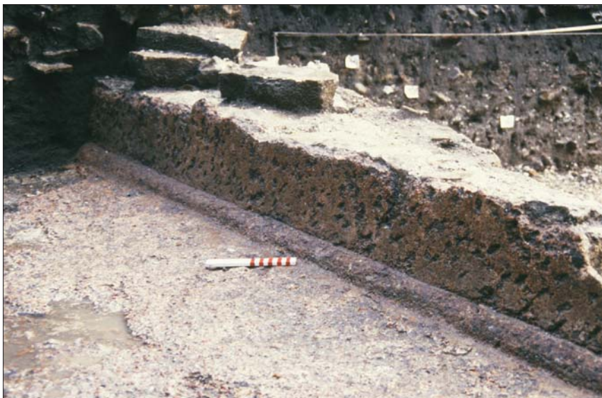
Figure 60: Building 8 showing the concrete lining
