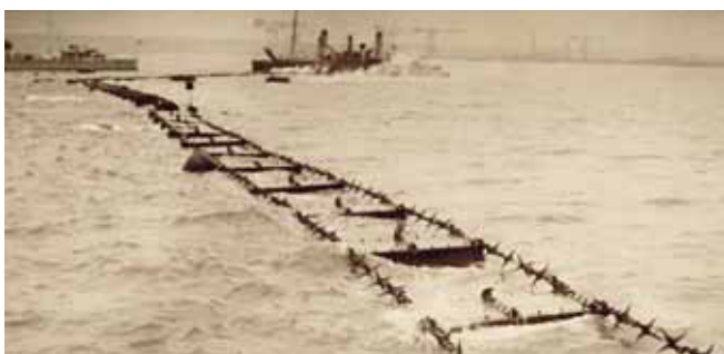
Figure 45: Submarine boom in place
