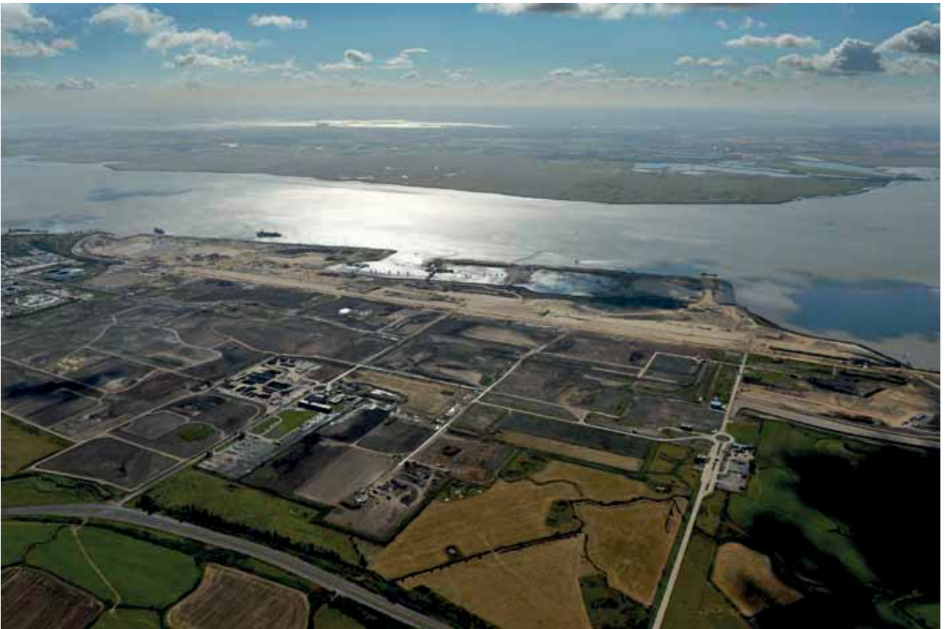
Figure 55: Aerial view of London Gateway port site
