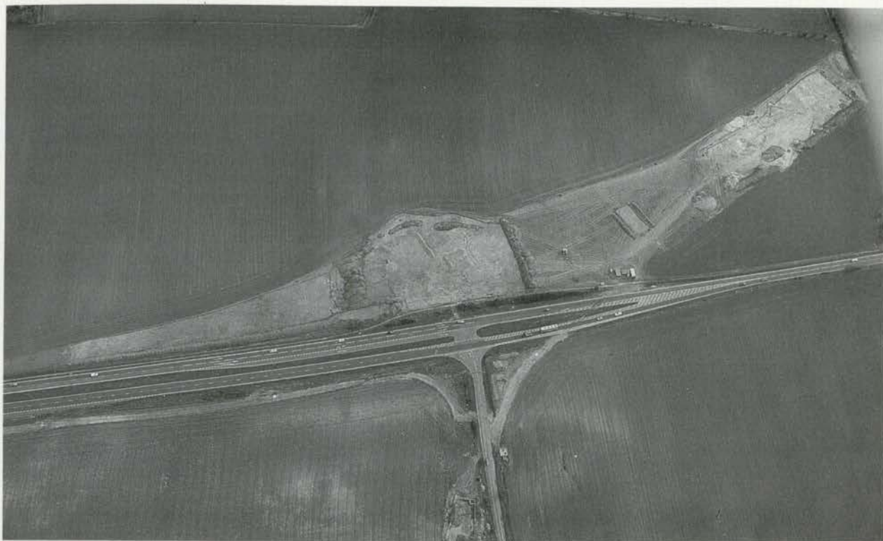
Plate 2 An aerial view, from the north, of the eastern end of the A27 Westhampnett Bypass route, with Area 2 in the centre. Areas 1, 3, 7, and 8 are also visible. Reproduced by permission of Steve Patterson
