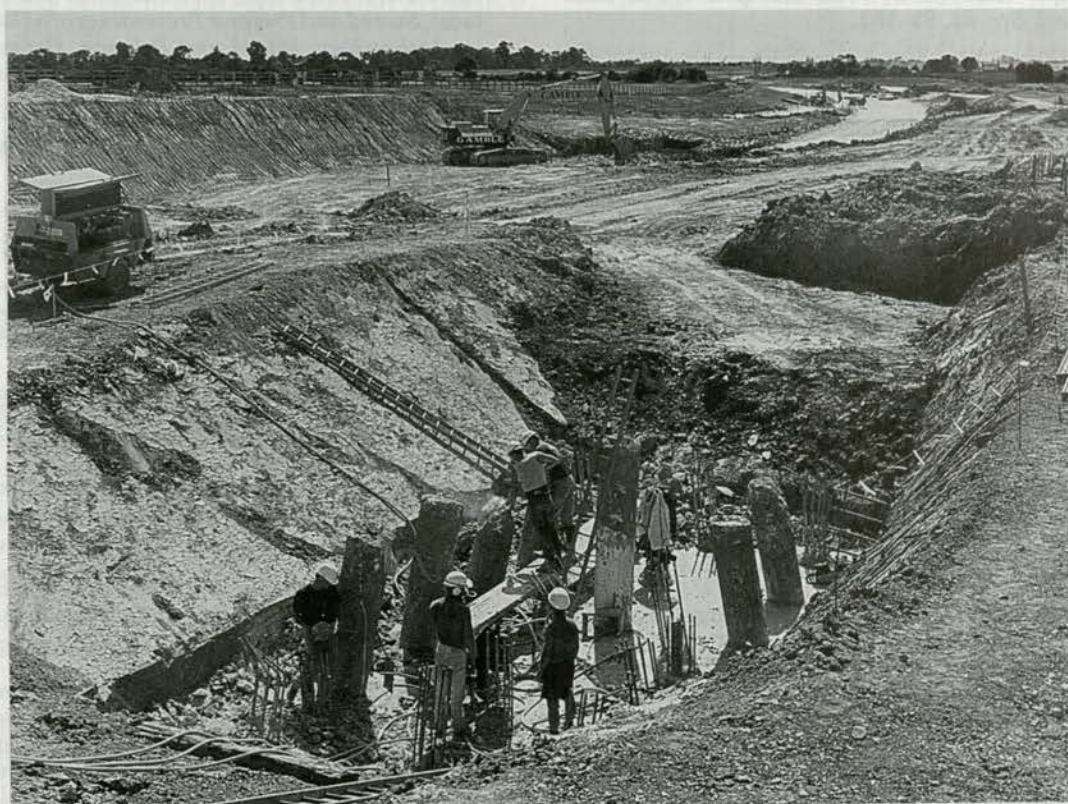
Plate 34 Area 2 during construction of the Bypass
