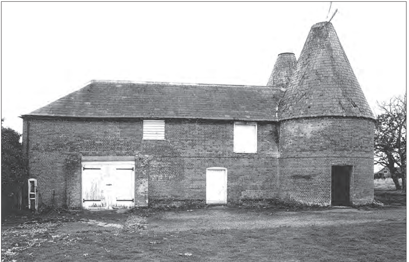
Figure 7.36 Yonse Farm: photograph of north elevation of double oast
