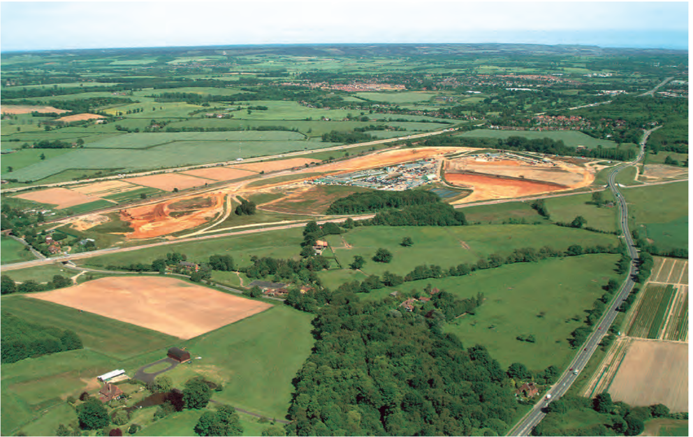
Figure 4.3 Beechbrook Wood Railhead under construction
