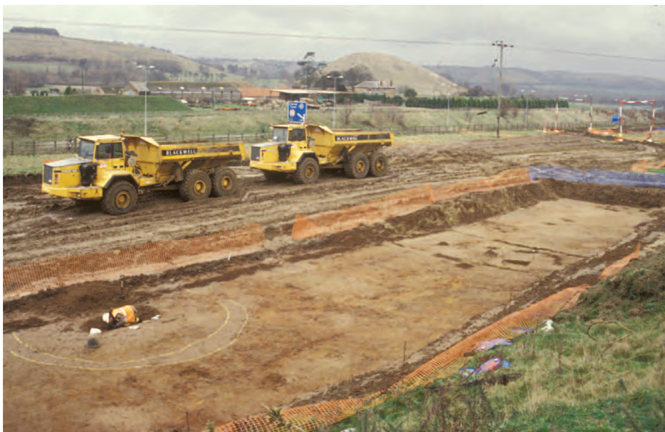
Figure 1.3 Saltwood tunnel: archaeology and construction work progressing in parallel
