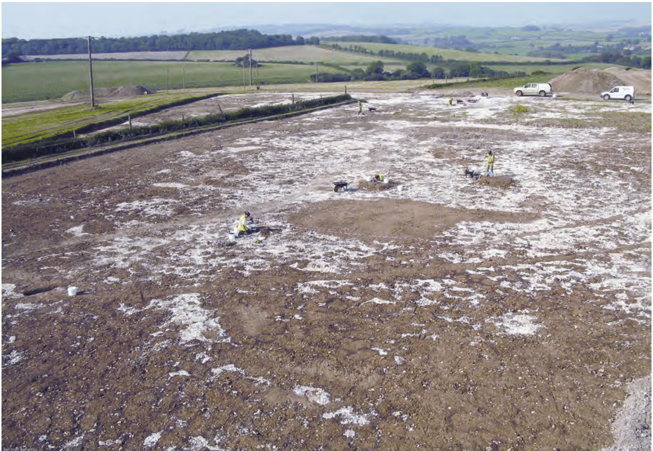
Plate 1.1 Excavation of Area 4 with probable Romano-British quarry in foreground
