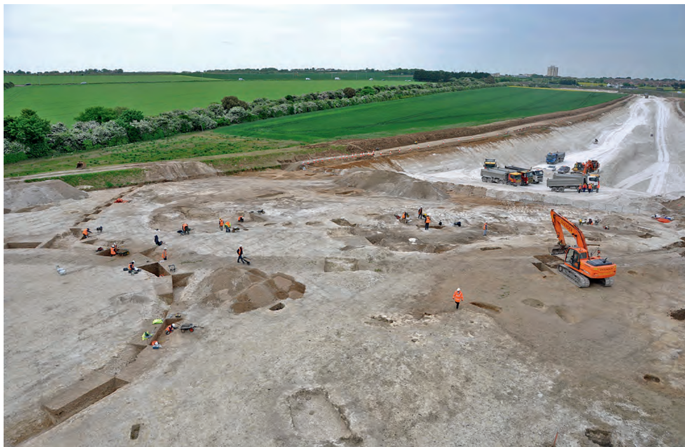
Pl 0.3 Excavations in progress in Zone 13, immediately ahead of tunnel approach works (view from west)
