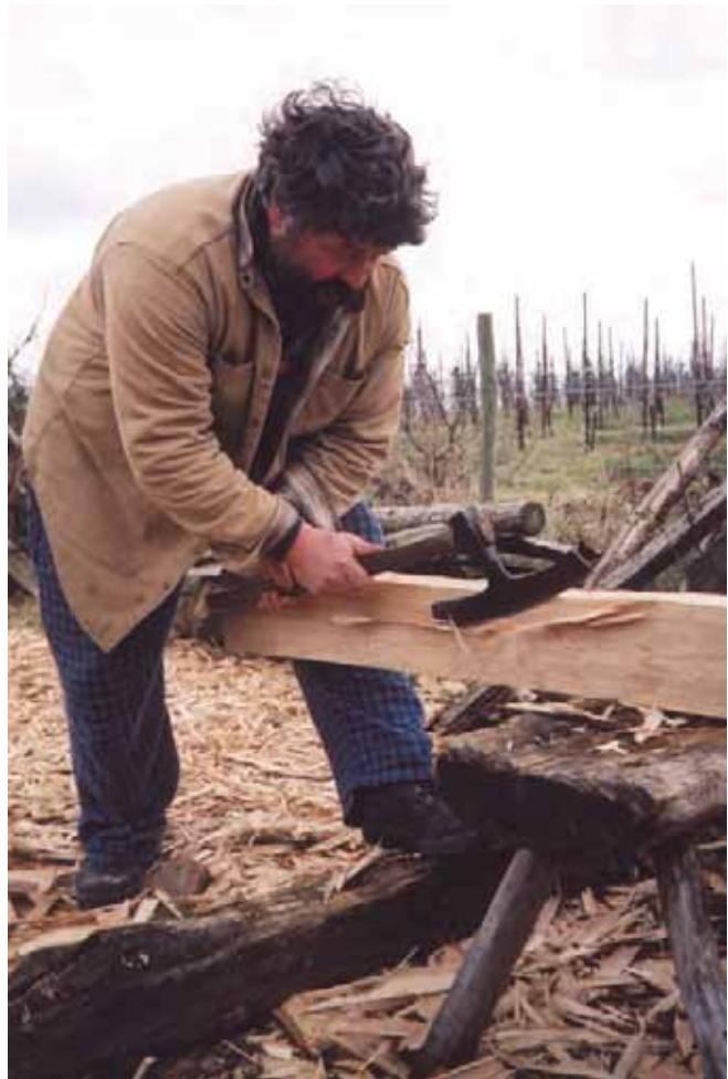
Plate 6.12 Smoothing an oak beam with a replica Saxon T axe, as used to create planks and piles for the mill
