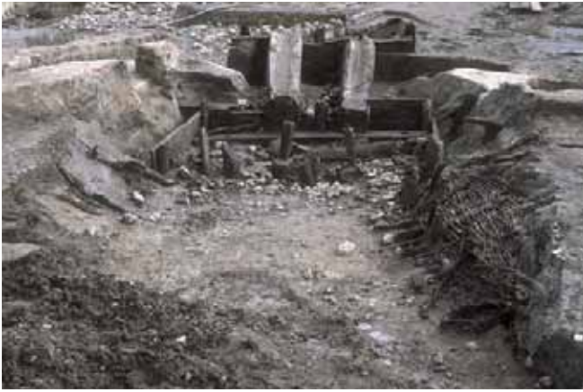
Plate 6.2 The tailrace and undercroft from the contemporary Ebbsfleet channel
