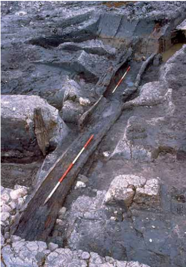
Plate 6.8 The mill pond spillway. Looking north
