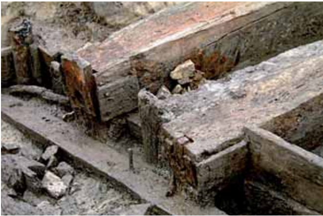
Plate 6.5 The pentrough outlets. Looking north-east
