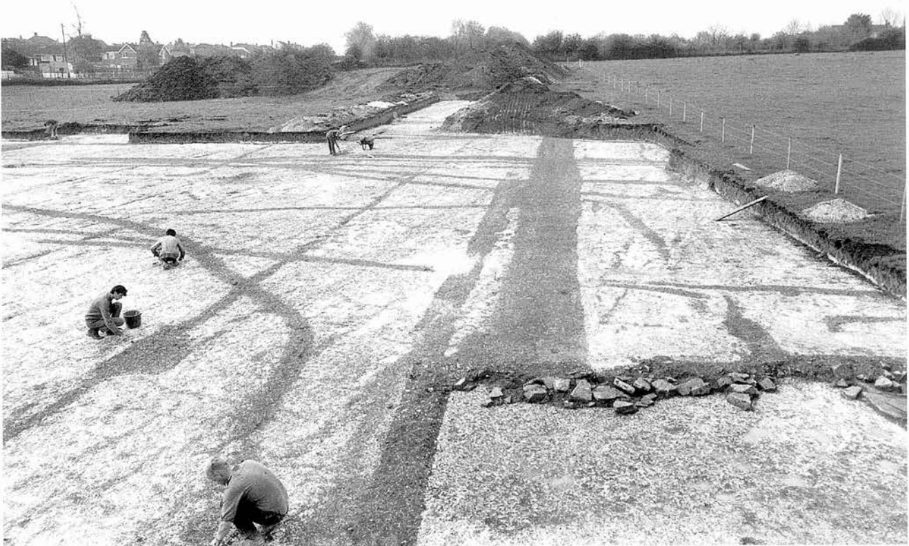
Figure 15 St Georges Road: western part of the excavation looking south; Period 6D medieval structure 01009 in foreground
