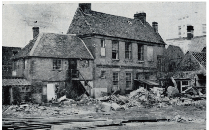
View of No. 25 from south during demolition, showing brick wing
