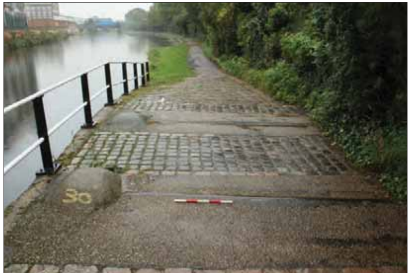
Plate 6.28: Tipping Wharf 1 with crane rails and concrete buffers (BHA 6)
