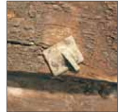
Copper rove bent over
