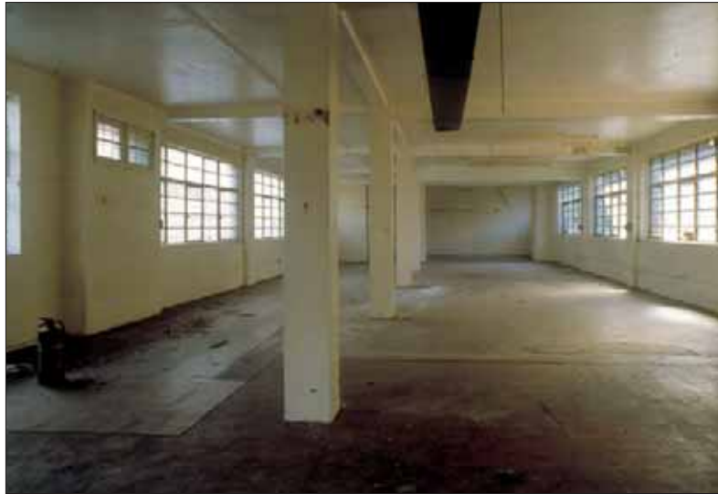
Plate 6.32: Interior of Robinson, King and Co's 1952 works building (BHA 13)
