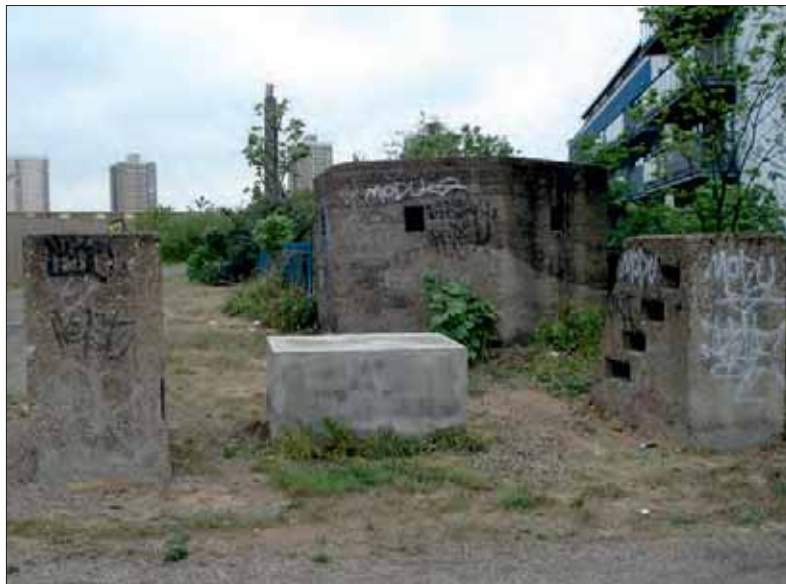
Plate 9.3: Tank block at Old Ford
