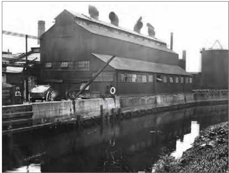
Industrial shed and adjacent building, Marshgate Works (BHA 4)
