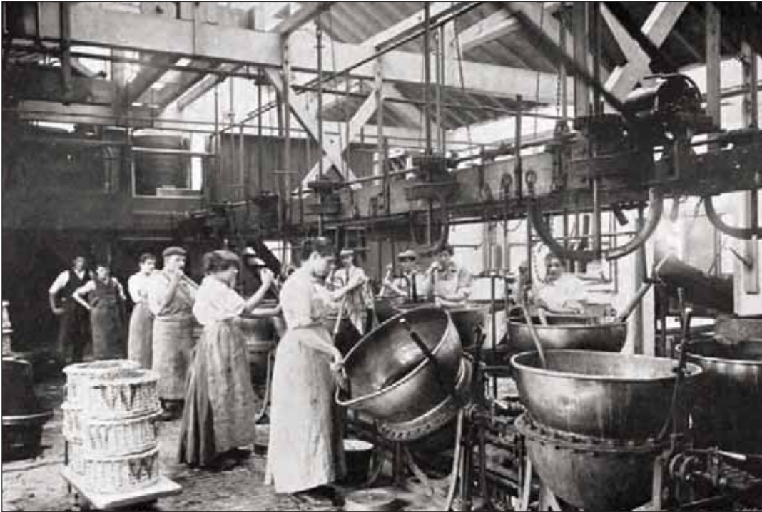
Plate 6.16: Employees in Clarnico's Jam Boiling Room (BHA 5)
