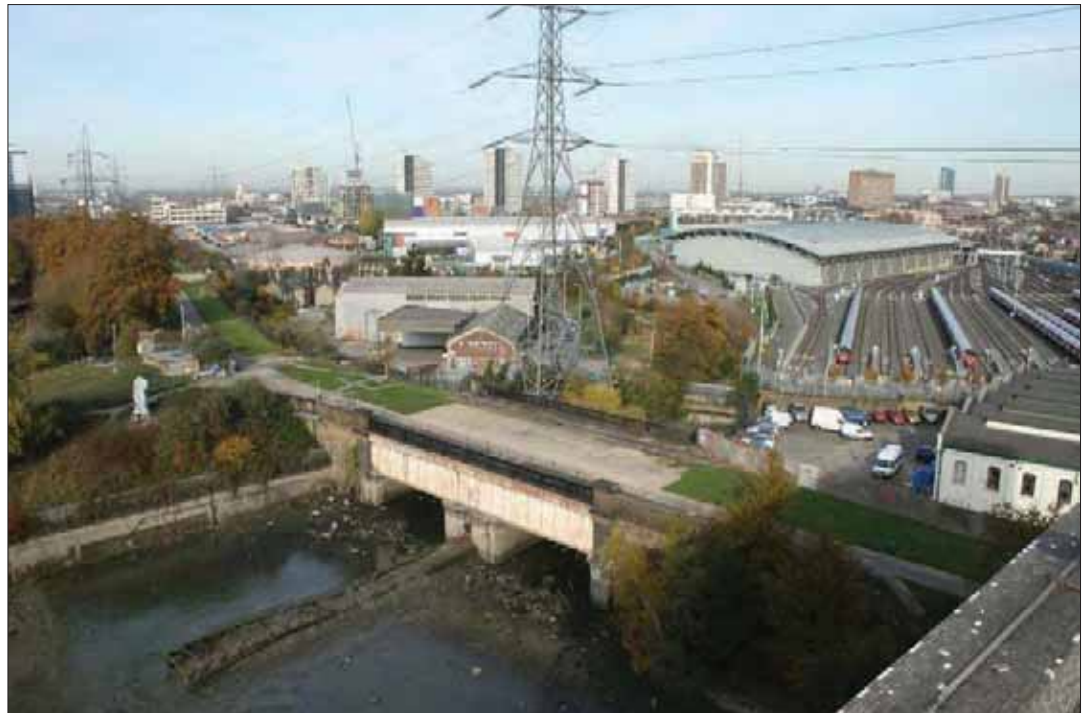
Plate 6.1: Bridge carrying the Northern Outfall Sewer across the Channelsea River
