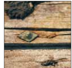
Copper rove and iron nail
