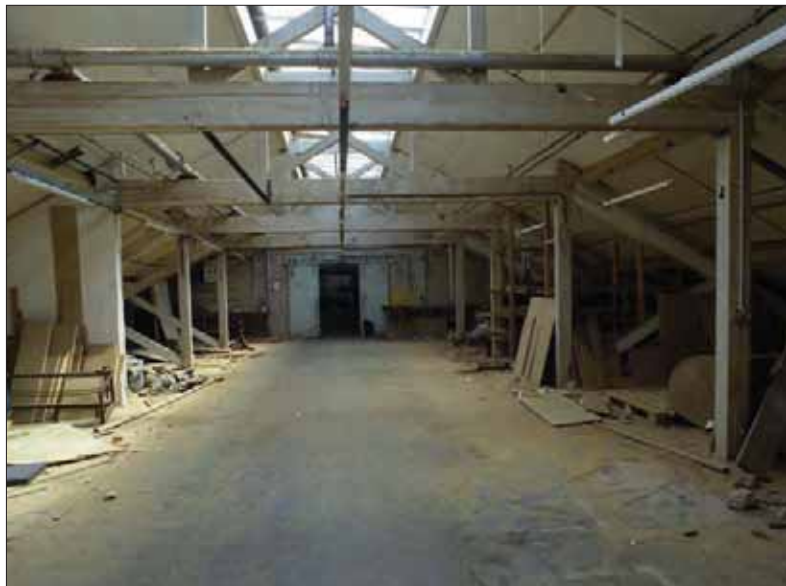
Plate 6.15: Internal view of queen post trusses of Clarnico's Starch Department (BHA 5)
