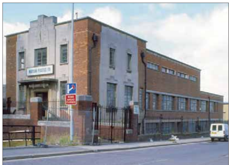
Plate 6.31: Exterior of Robinson, King and Co's Offices (BHA 13)
