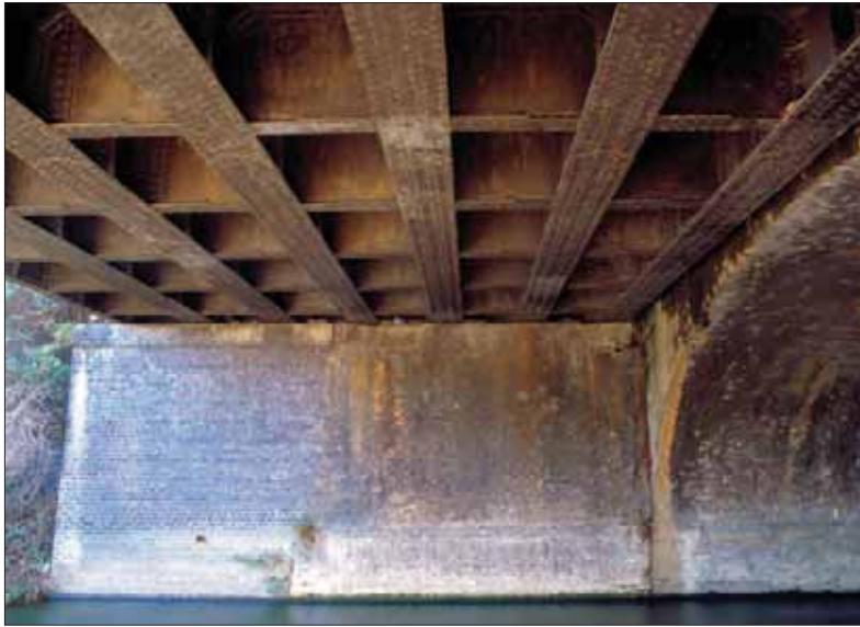
Plate 6.23: The widening of the GER bridge over City Mill River (BHA 36)
