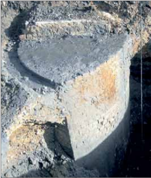
Plate 5.7: Prow-shaped brick pier base of compensation reservoir intake/discharge gate, Trench 61, from the west
