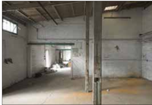
Plate 6.17: Interior view of the Clarnico stables (BHA 5)
