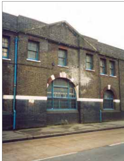
Plate 6.19: Central pedimented element of Yardley's building Y5 (BHA 23)
