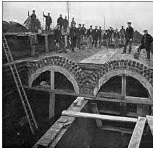
Plate 6.2: Additional pipes of Northern Outfall Sewer under construction
