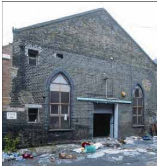
Plate 6.10: Exterior of Unit 6a, Vanguard Estate (BHA 15)
