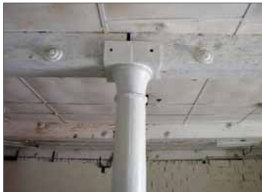
Plate 6.8: Ground floor cast-iron column and flitched joist, Unit 1, Vanguard Estate (BHA 14)
