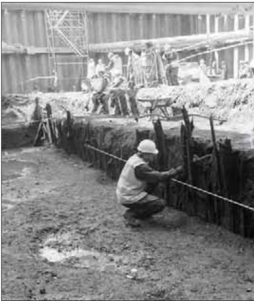
Plate 6.5: Phase 4 revetment of Tumbling Bay Stream in Trench 75, from the north-east
