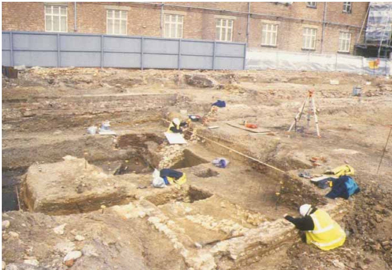
Figure 38: Excavating the foundations of a series of medieval buildings constructed over the edge of the infilled channel.
