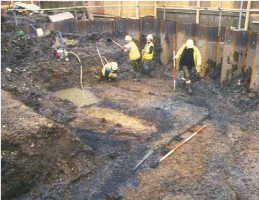
Figure 97: 16th and 17th century revetments in Trench 1a prior to excavation.
