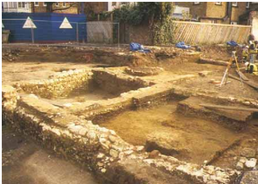
Figure 52: Foundations and bottom courses of a late 15th century building at 90° to Emms Passage – perhaps a precursor to the later maltings in this property.
