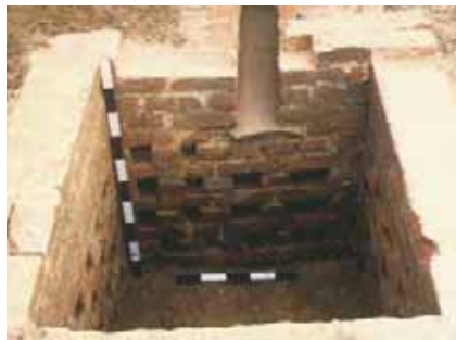
Figure 67: Brick-lined soakaway. This contained a deposit of animal bones—perhaps waste from tanning or leather working.
