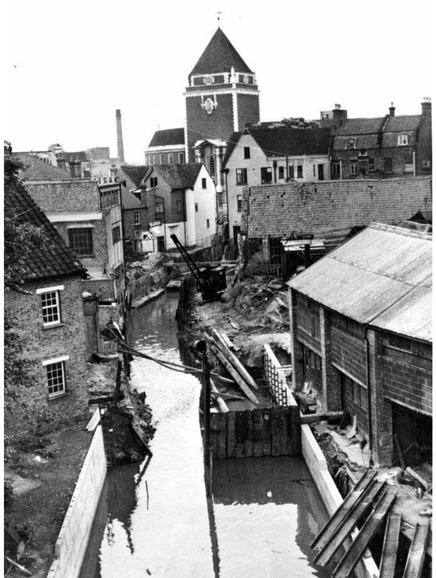
Widening the Hogsmill in the 1950s.
