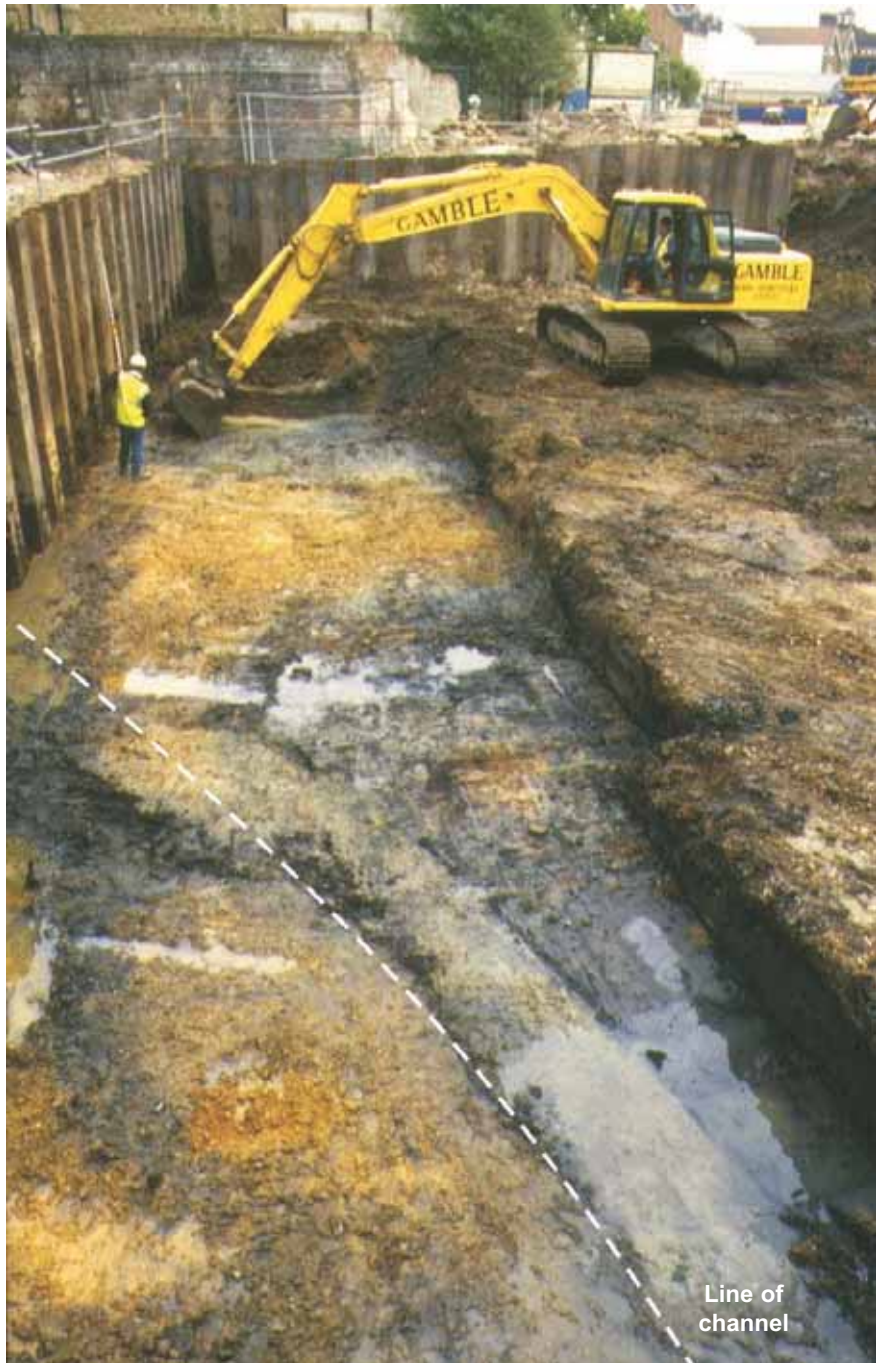
Figure 7: Silts being removed down to natural gravel in the Hogsmill channel. The parallel lines of two 13th century timber revetments can be seen extending from the bottom right.
