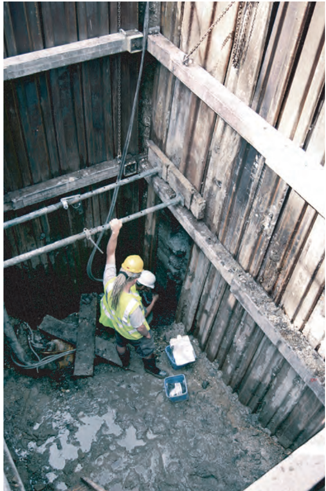
Plate 13.1 Trench 9 shored trench excavation
