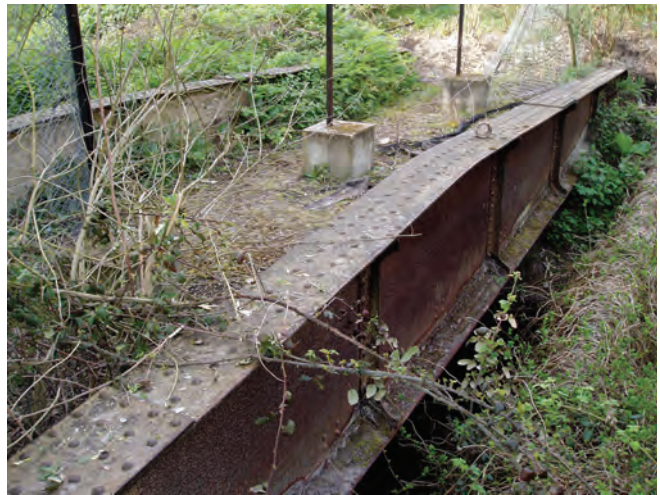
Plate 2.1 Late 19th-century pit-rail rivet bridge across the Ebbsfleet into Baker's Hole and Southfleet Pit
