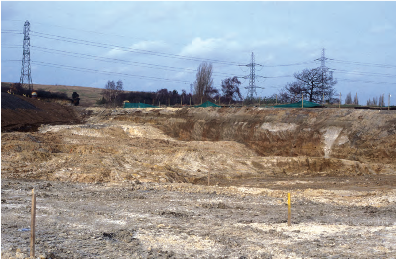
Plate 10.8 Main section in the Jayflex remediation area
