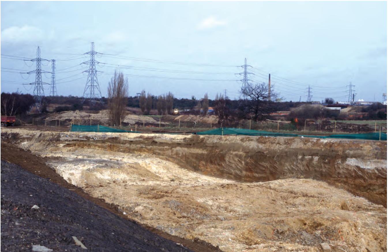
Plate 10.9 Western end of section in the Jayflex remediation area
