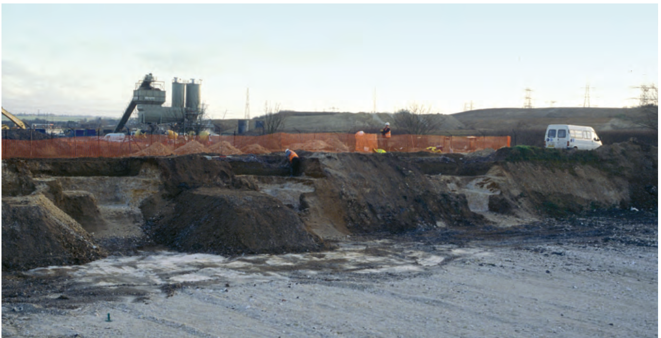
Plate 9.1 View of 4018TT, 4019TT and 4020TT, excavated and cleaned
