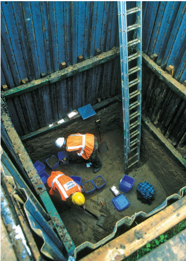
Plate 5.1 3776TP, excavation shoring
