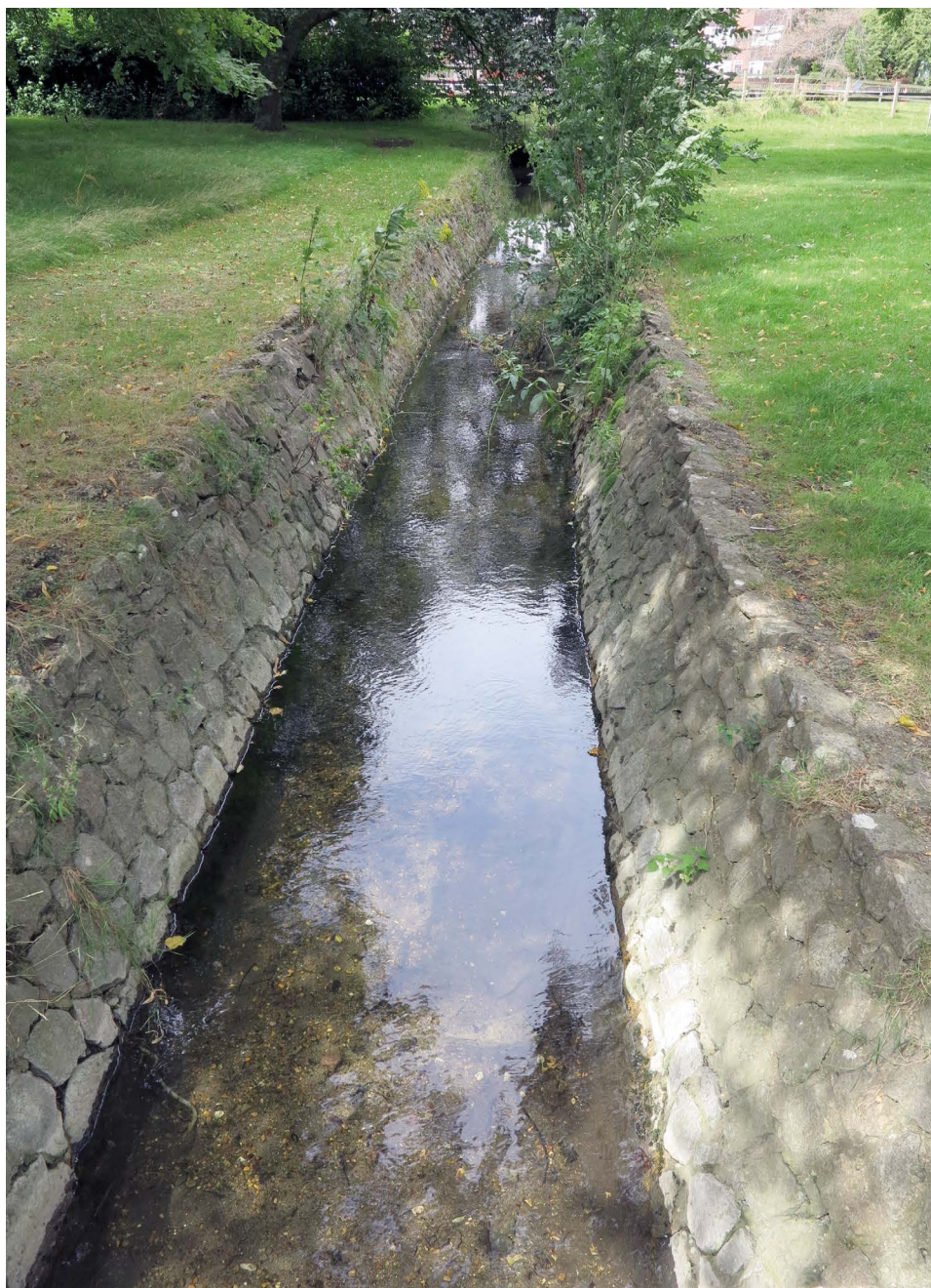
Plate 4.11 Modern water channel in Churchill Gardens, of probable similar dimensions, construction and appearance to the medieval Town and Close Ditches
