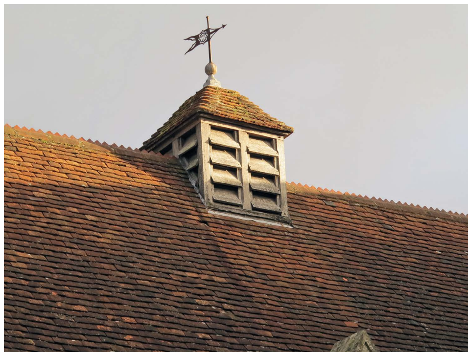
Plate 4.17 The Medieval Hall, Cathedral Close: cockscomb ridge tiles would once have been a familiar feature of the city skyline, as would louvers before the gradual introduction of chimneys
