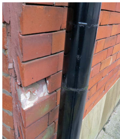
Plate 4.30 Windover House, St Ann Street: mathematical tiles of the 19th century, showing (top) facade, (left) construction and (right) junction with brick construction
