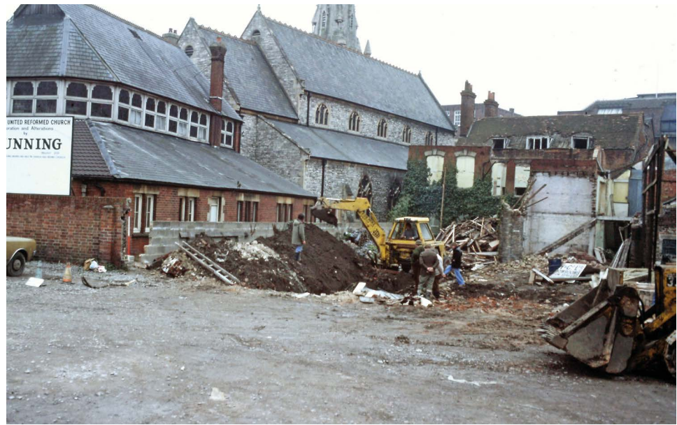
Plate 2.4 The Maltings: rescue excavations in 1978, showing general location
