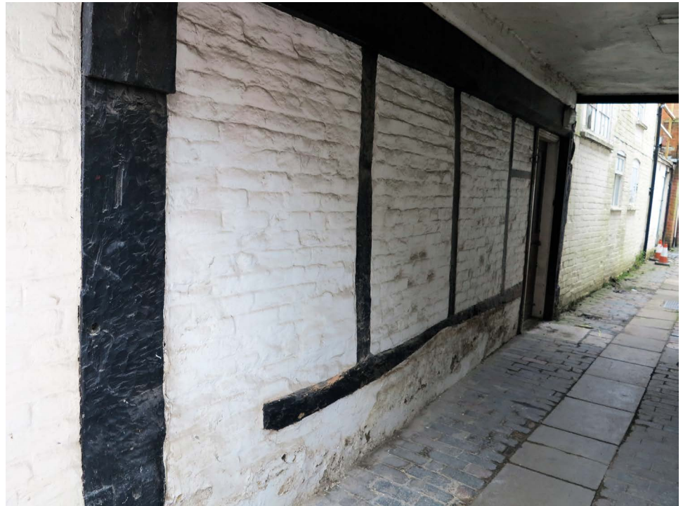
Plate 4.19 Building width, possibly based on a perch, as seen in No. 63 Castle Street, early 16th century
