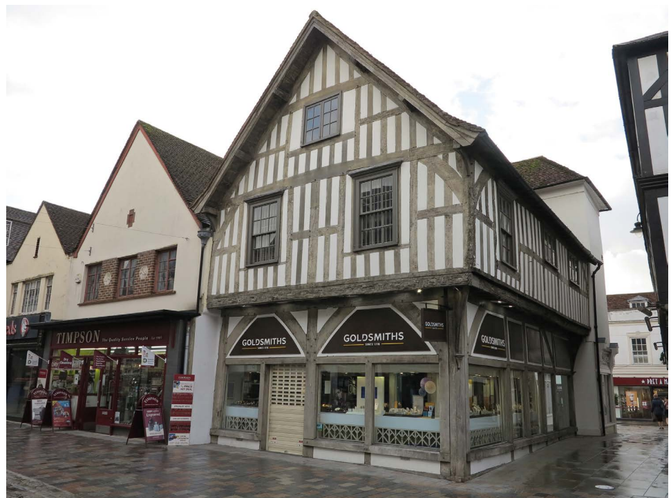
Plate 4.21 Medieval buildings with length=twice width with gable facing the street: No. 33 Butcher Row, similar design and dimensions, probably 15th or 16th century
