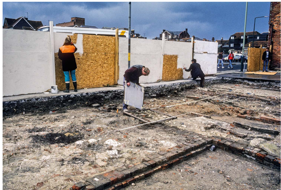
Plate 2.20 Brown Street (W227): general view of work at the street frontage from the south-east
