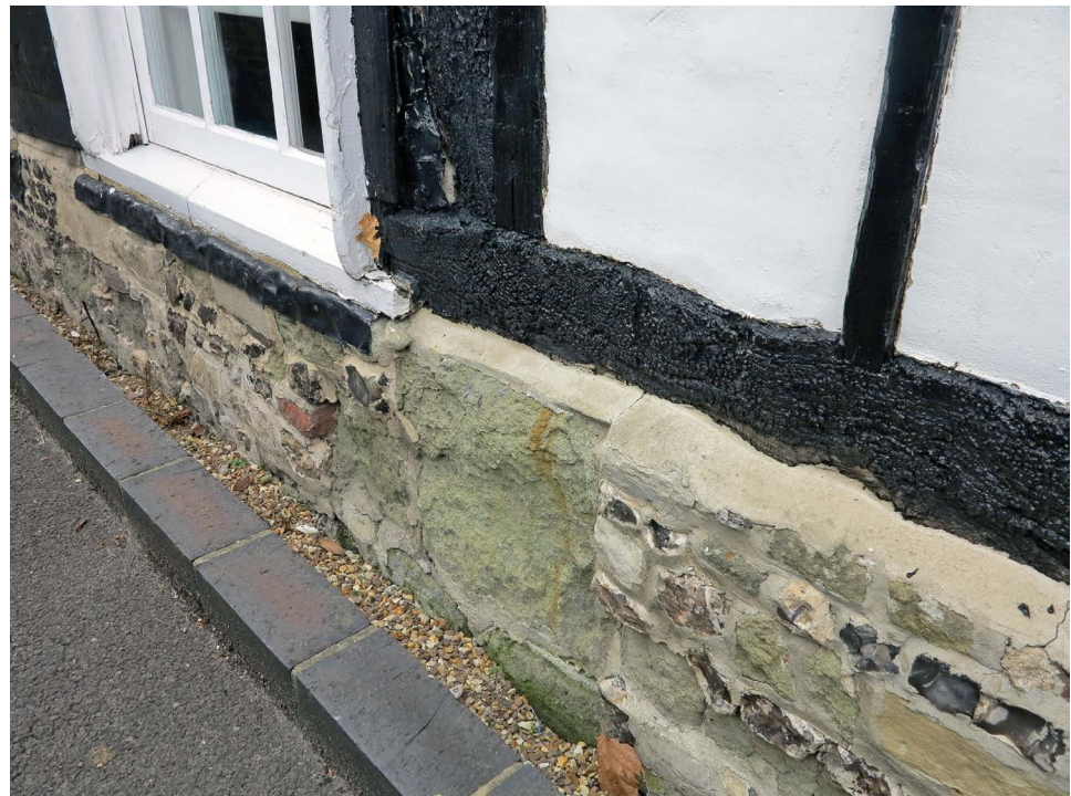
Plate 4.18 Greensand block supporting vertical member of timber-framed building
