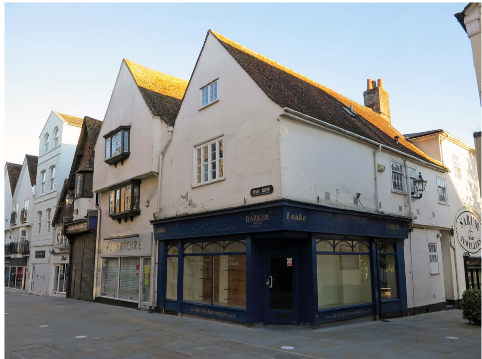
Plate 4.20 Medieval buildings with length=twice width with gable facing the street: Wheatsheaf Inn, Nos 7–9 Fish Row, 14th century
