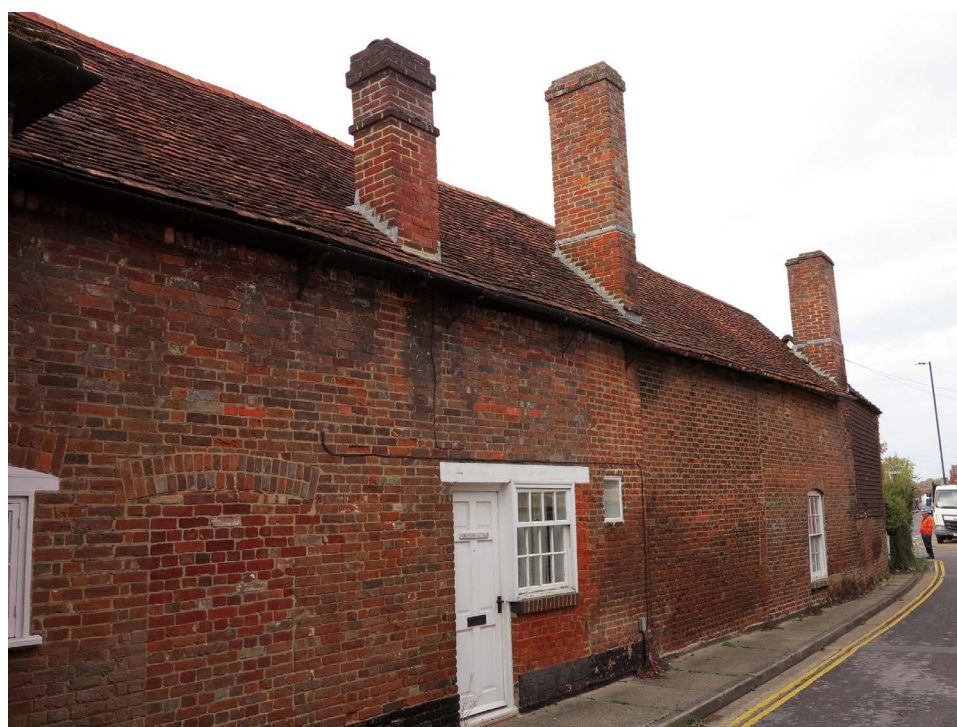
Plate 4.27 Showing chimney on the street frontage: examples off St Ann Street
