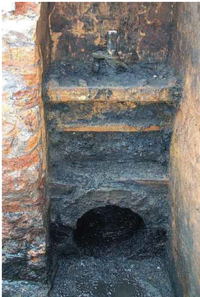
Fig. 17 The valve assembly in the sluice chamber
