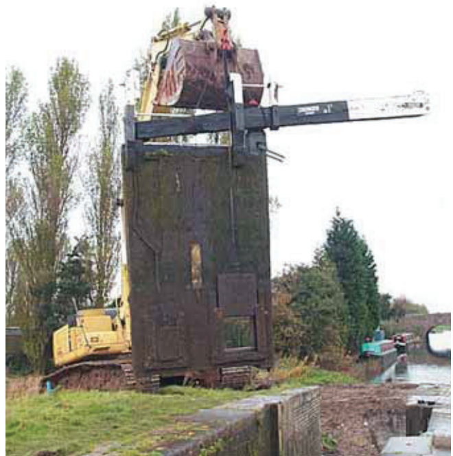
Fig. 194 Reclamation of the lower lock gate
