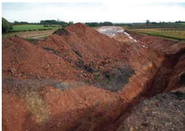
Fig. 51 Section through the canal and embankment viewed from the north-west
