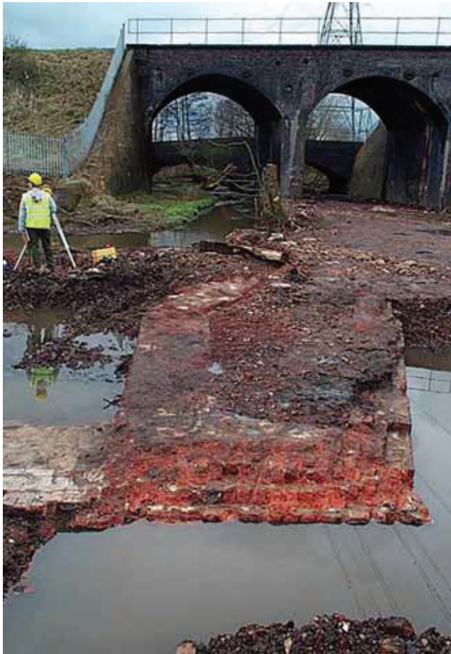
Fig. 22 The western side of the basin entrance looking west towards the railway and accommodation bridges
