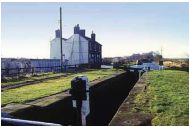
Fig. 188 View of the lock and cottage from the north-east
