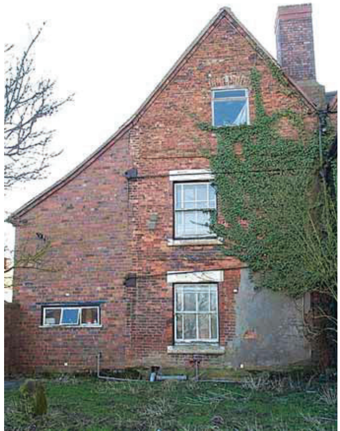
Fig. 38 The west elevation
