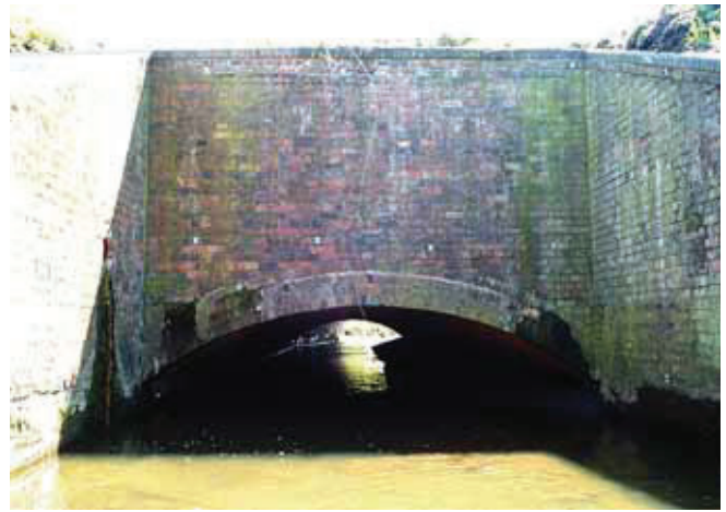
Fig. 19 The culvert carrying the embanked canal aqueduct over Wyrley Brook
