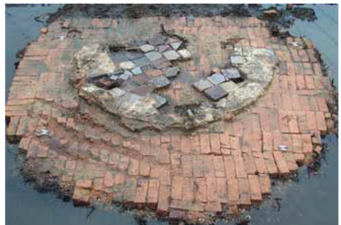
Fig. 26 The crane base
