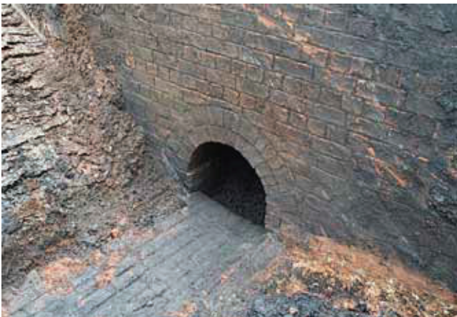
Fig. 15 The arched opening of the drain in the canal basin
