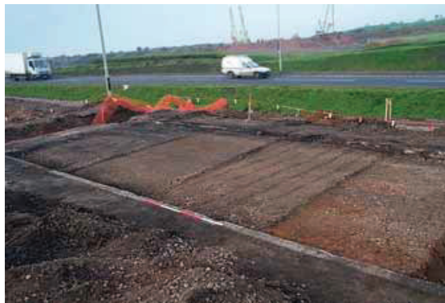
Fig. 48 Plough scars in the old road surface
