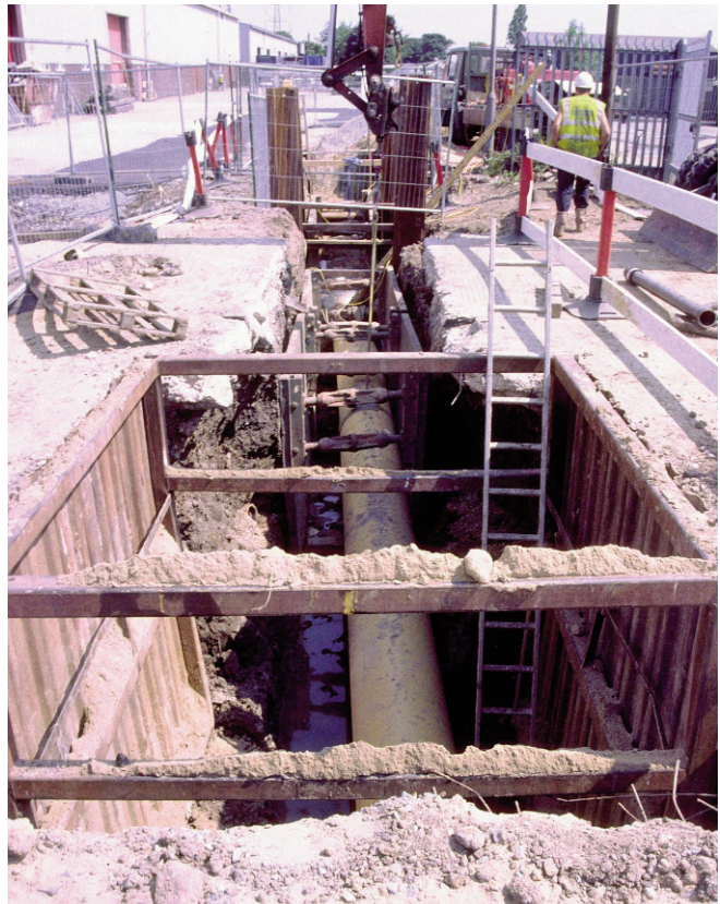
Plate 12 Pipeline excavations employing box shoring through the Ford Motor Works
