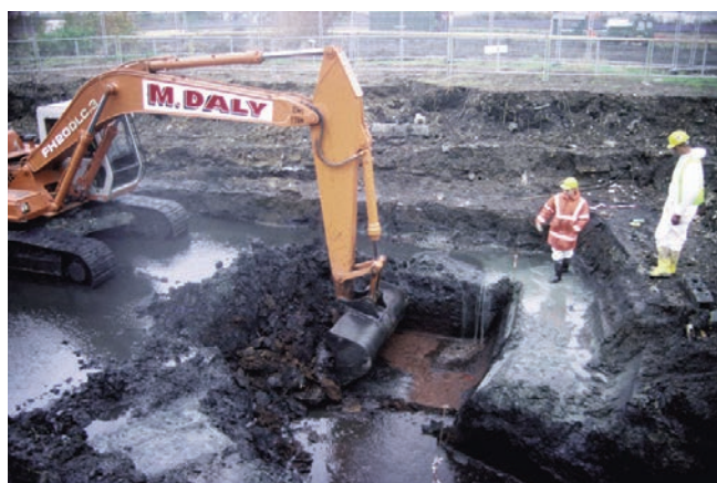
Plate 10 Excavations at the Goresbrook diversion
