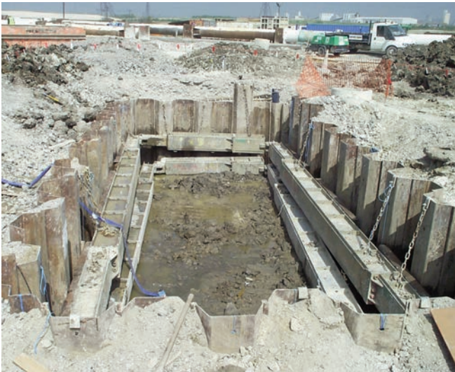
Plate 22 Cofferdam excavation 3880TT, Swanscombe
