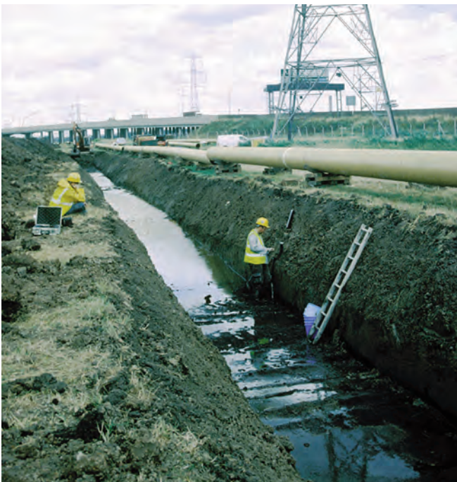
Plate 14 Open trench pipeline excavations on Rainham Marsh
