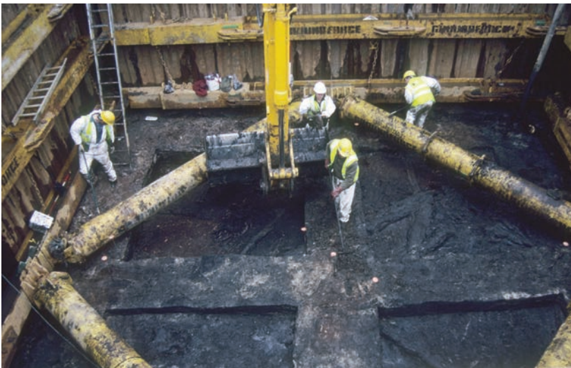
Plate 29 Area 4 cofferdam excavation in the Ebbsfleet Valley (STDR4 01)
