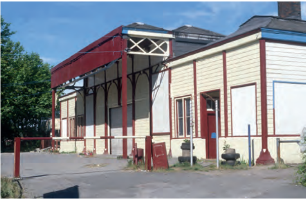
Plate 17.12 LMS railway station, Oxford, copyright OA
