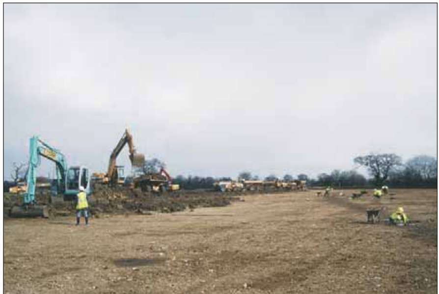
Plate 1.1: The scale of the excavations - removing topsoil on the LTCP site
