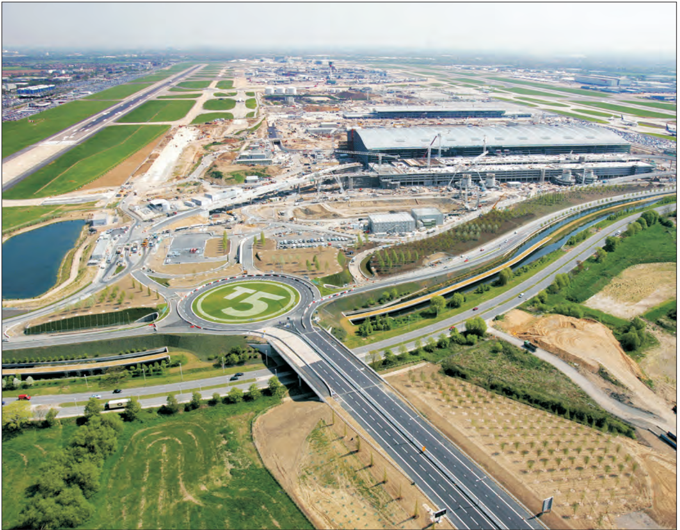
Plate 1.1: Heathrow Airport, aerial view of T5 construction site, May 2006 (© BAA Limited see www.baa.com/photolibrary )
