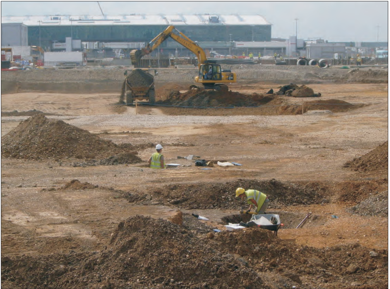
Plate 1.3: Working shot of excavations at Terminal 5
