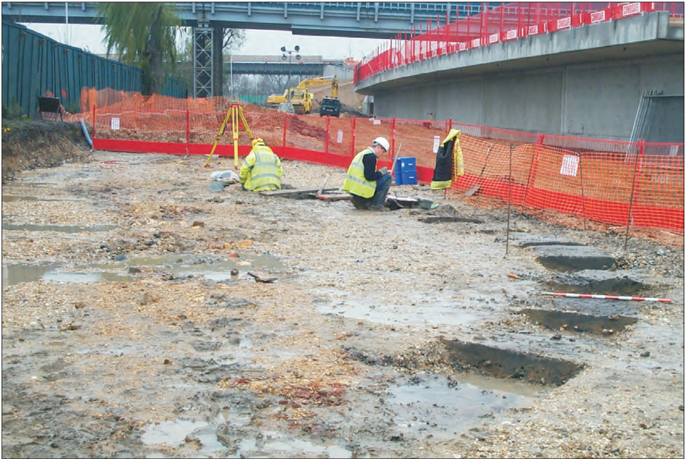
Plate 2.34: HE3 enclosure under excavation
