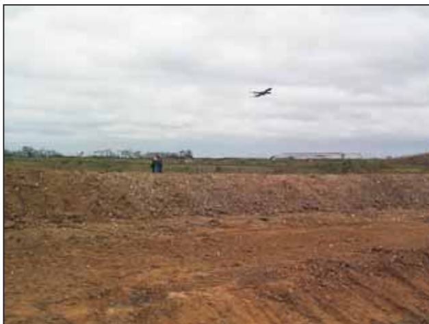
Plate 2.5: Reconstructed cursus central bank looking east
