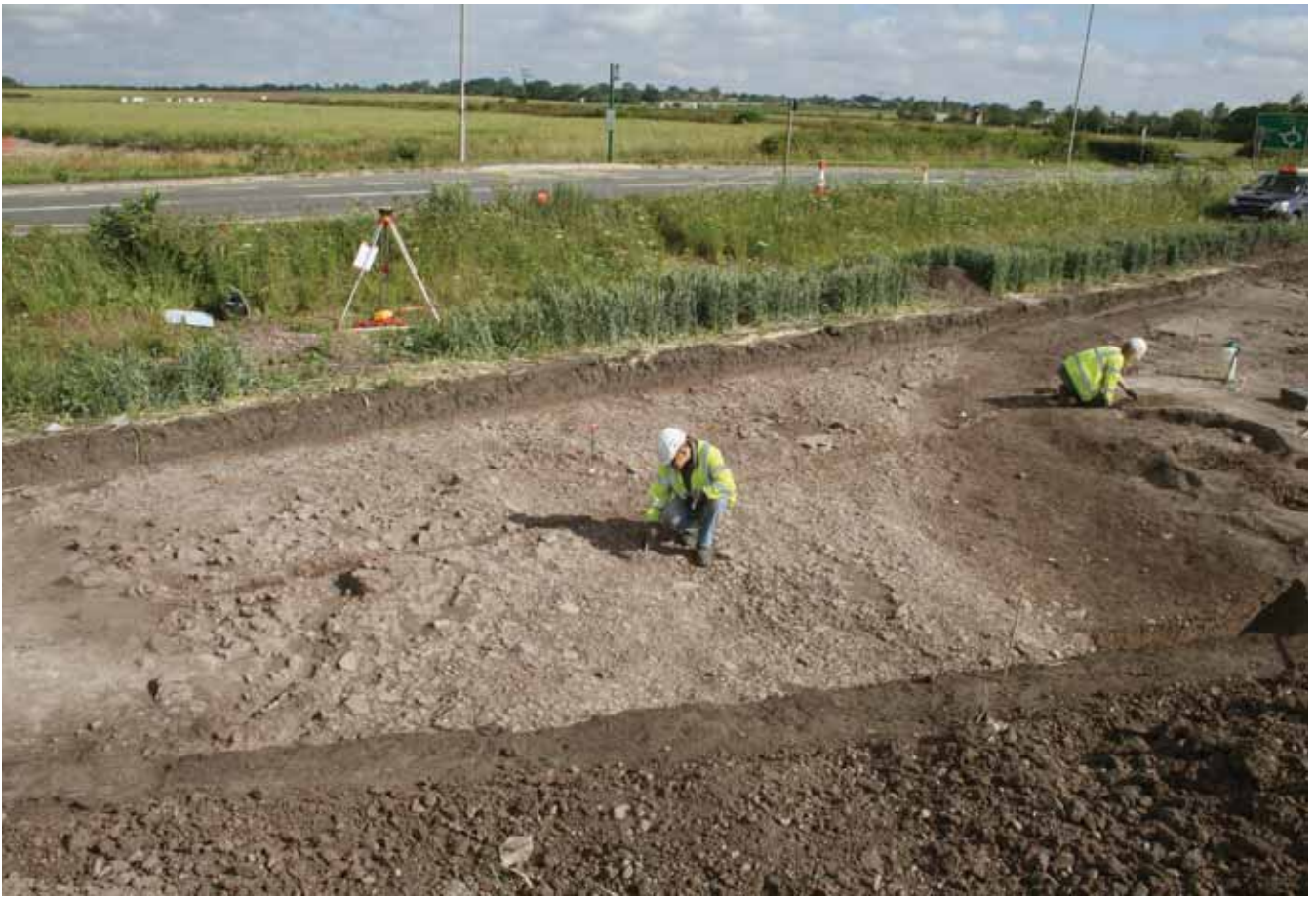
Fig. 4.47 Road 303505 under excavation, viewed from the south
