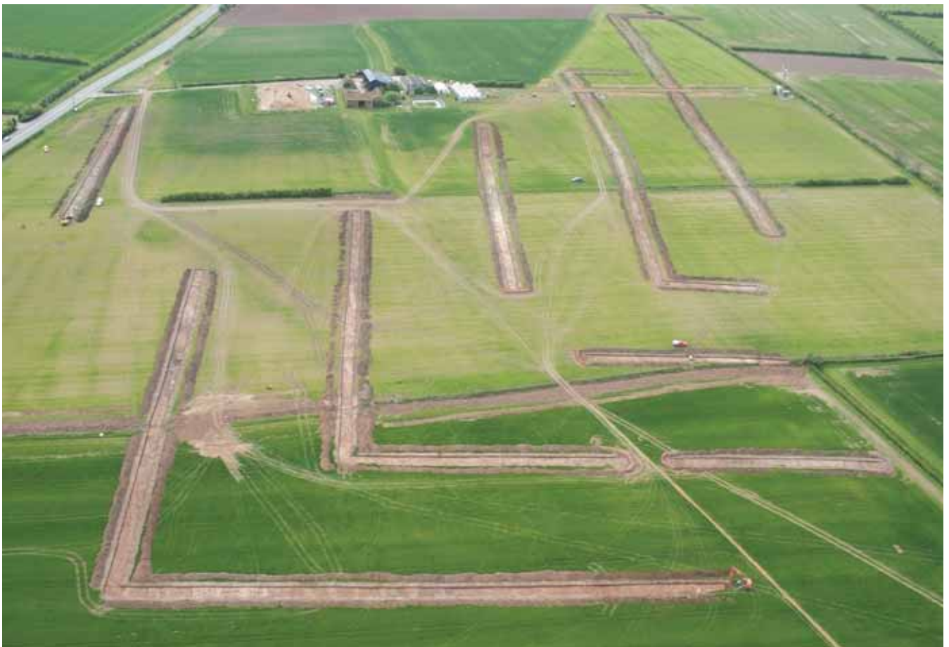
Fig. 1.4 SM trenches at Saxondale
