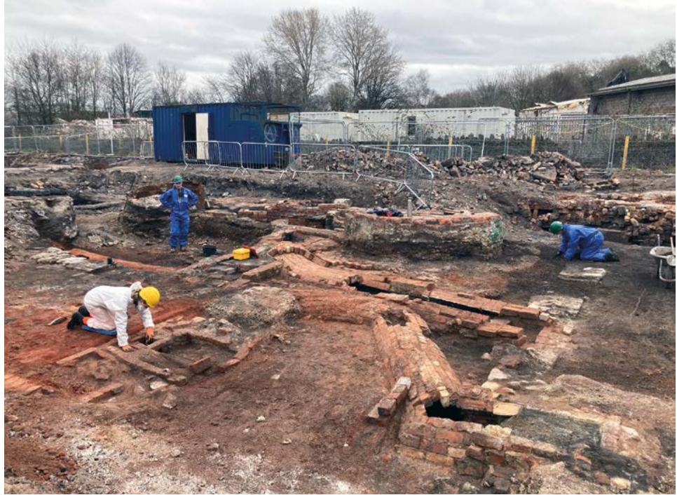
Figure 4.13 Buildings B1 and B6 and flues S11 and S21, looking north-east
