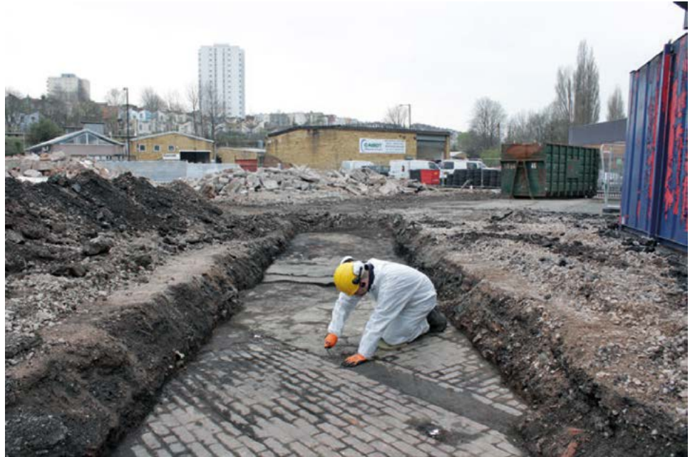
Figure 7.4 Floor of the Bedminster Iron Tomb Railing and Iron Foundry (B23), looking south
