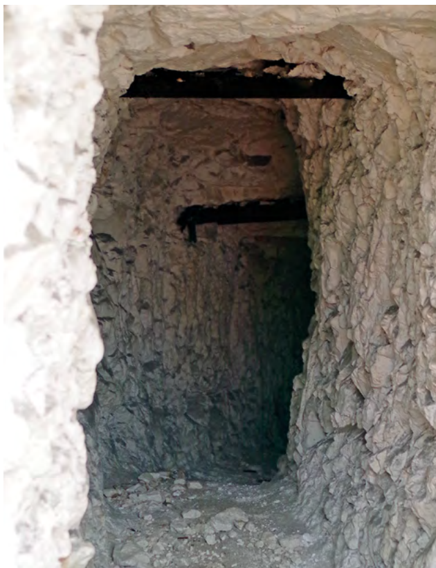
Figure 3.17 Wooden horizontal lintels to shore the roof of tunnel TG8
