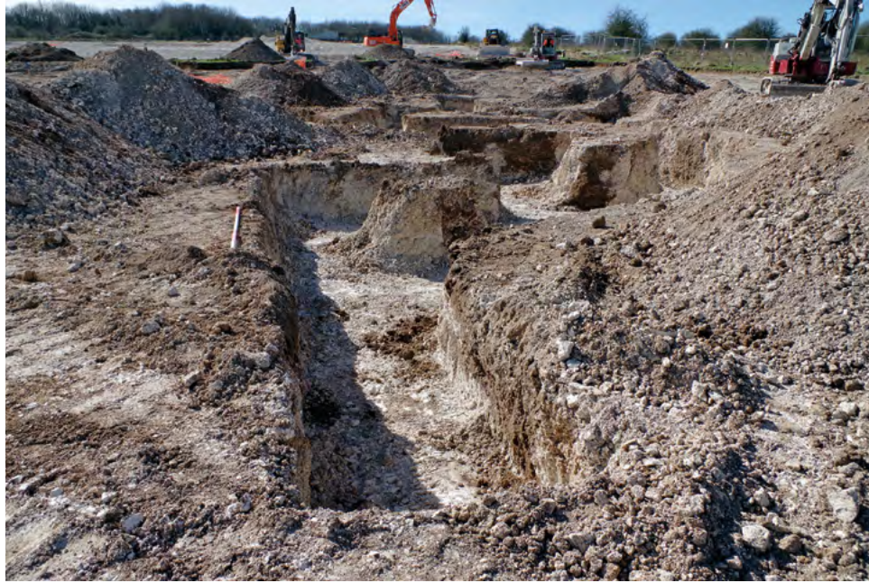
Figure 3.9 Blue Line Phase 1 crenulated fire trenches
