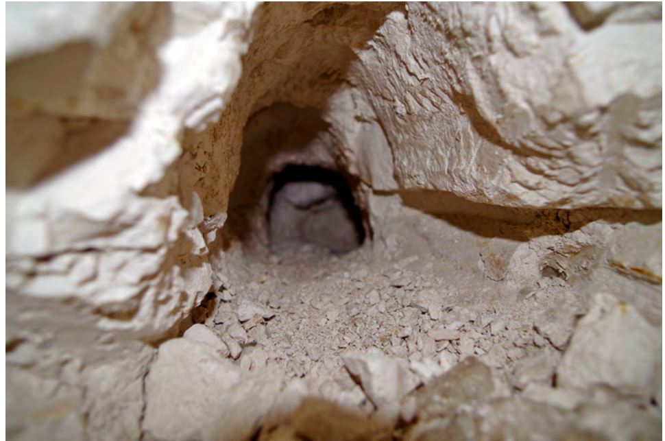
Figure 3.13 Hole for setting of torpedo camouflet charges TJ5 'j'
