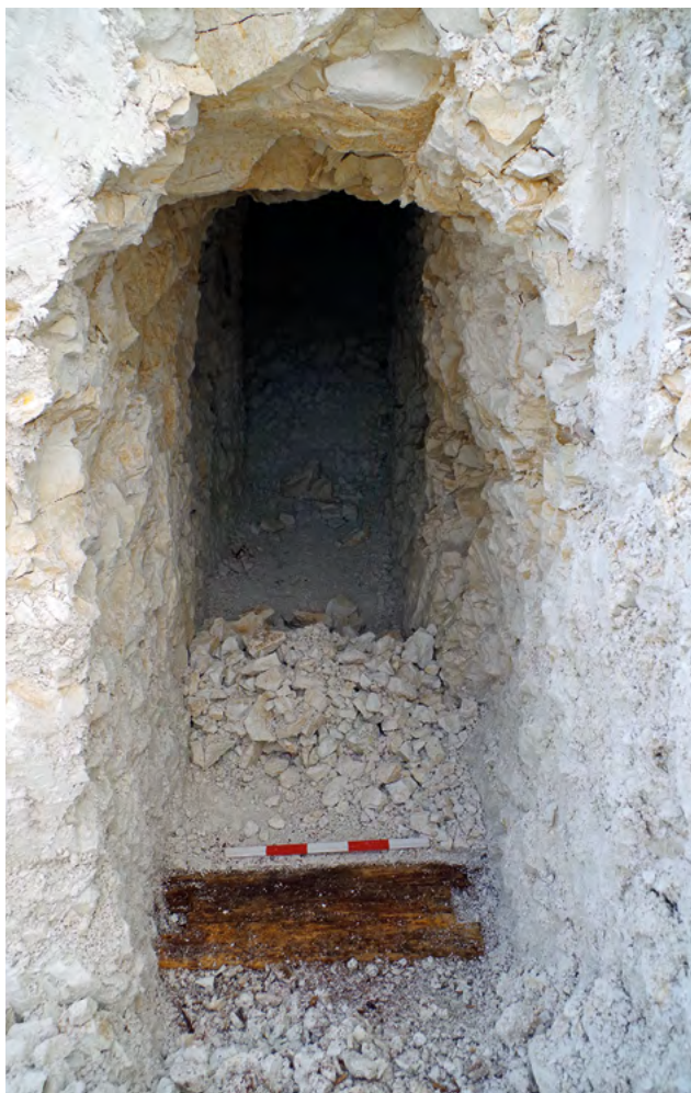
Figure 3.15 TF13. A horizontal timber plank with mortise holes in each end, interpreted as part of a frame for a gas curtain of treated canvas, designed to impede the ingress of poison gas underground
